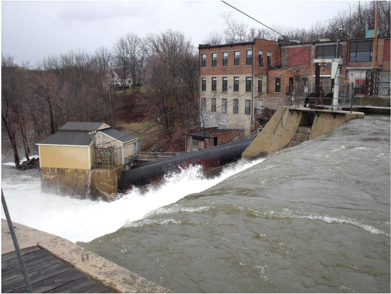
Figure 5 – Plant 9B Intake, Penstock, and Powerhouse
