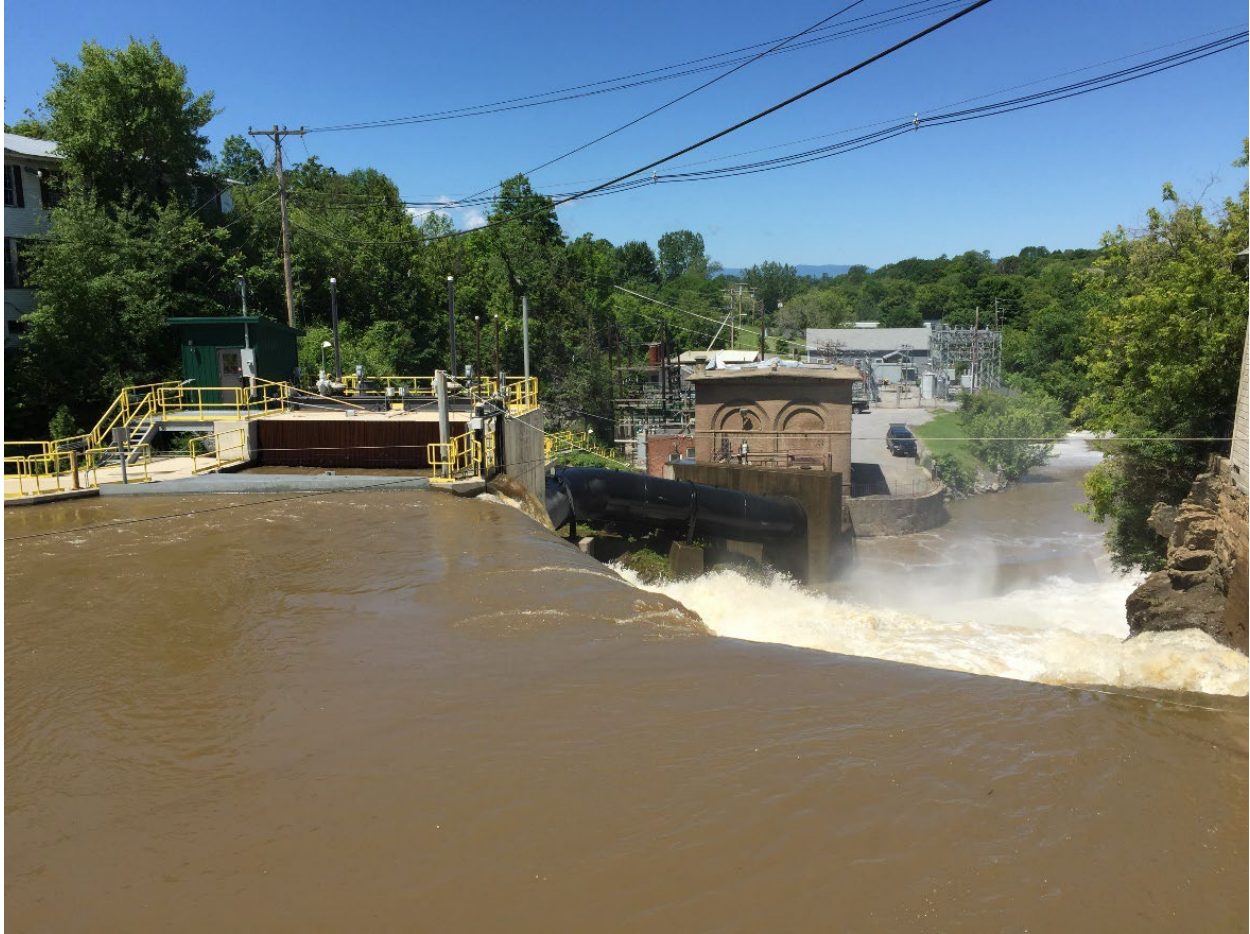
Figure 4 – Plant 9 Intake, Penstocks, and Powerhouse.
