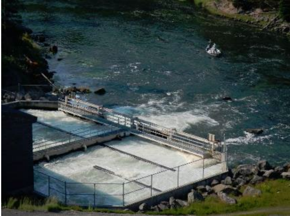
Figure 8 – Powerhouse Aeration Basin and Tailrace
