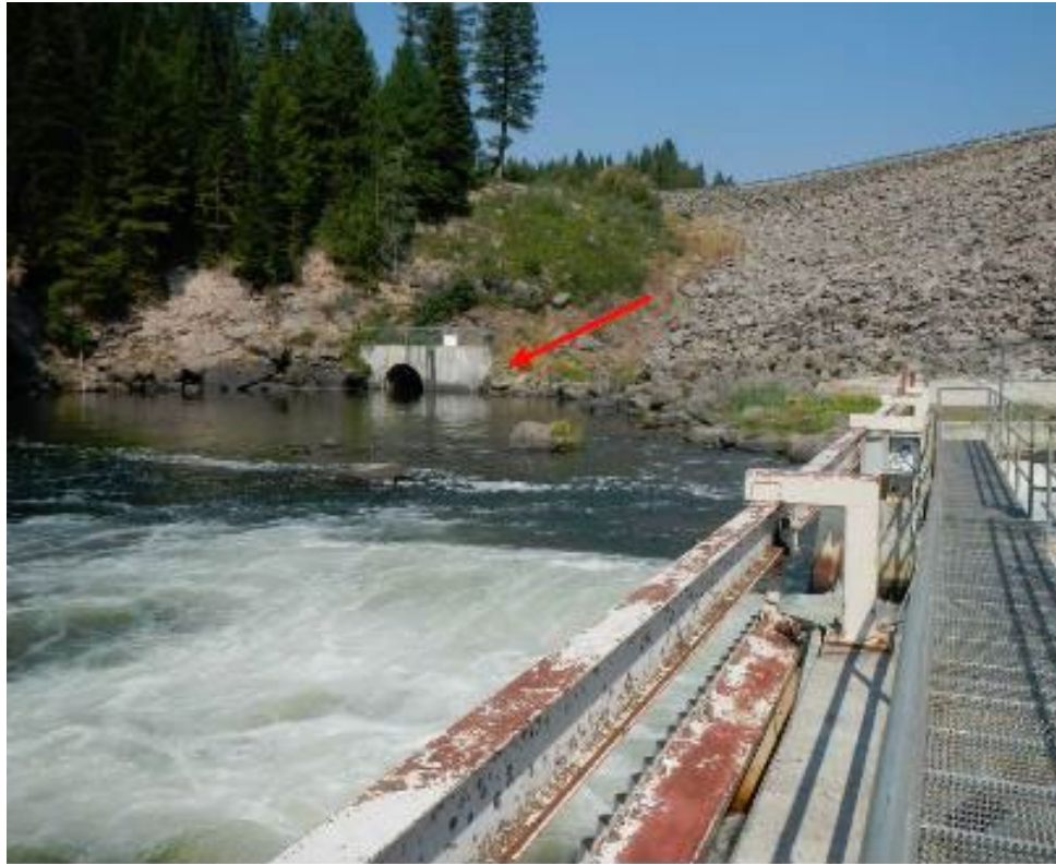
Figure 6 – USBR Tunnel Outlet
