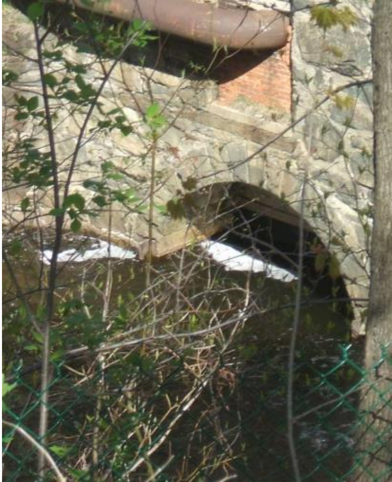
Figure 3. Stone Arch Discharge
