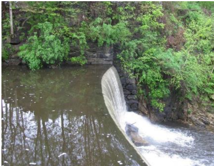
Figure 2. Project Dam and Spillway
