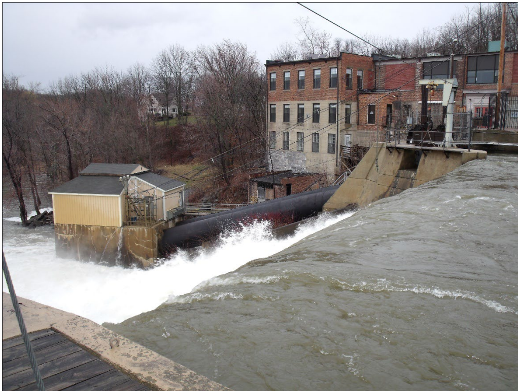
Photo 3 Plant 9B Intake, Penstocks, And Powerhouse
