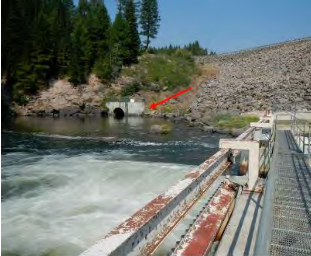
Figure 4. USBR Outlet Tunnel.
