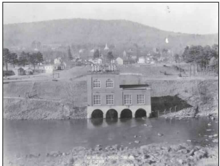
Deerfield No. 3 Development, Buckland/Shelburne, MA, built 1912 et seq. View of powerhouse looking south across Deerfield River from Shelburne Falls to Buckland (November 25, 1941 photo). View shows turbine outfall arches below powerhouse. Deerfield No. 3 was the administrative and maintenance center for the Lower Deerfield developments, and several of the workshops and storage buildings are visible behind the powerhouse to the left.
