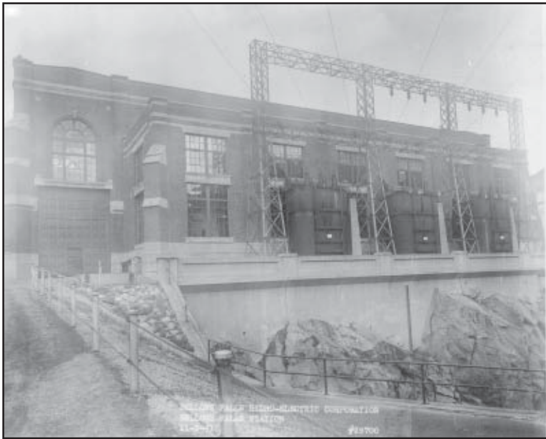
Bellows Falls Development, North Walpole, NH/Rockingham, VT, built 1925–1928. View of powerhouse looking north with transformers at right (November 3, 1941 photo).
