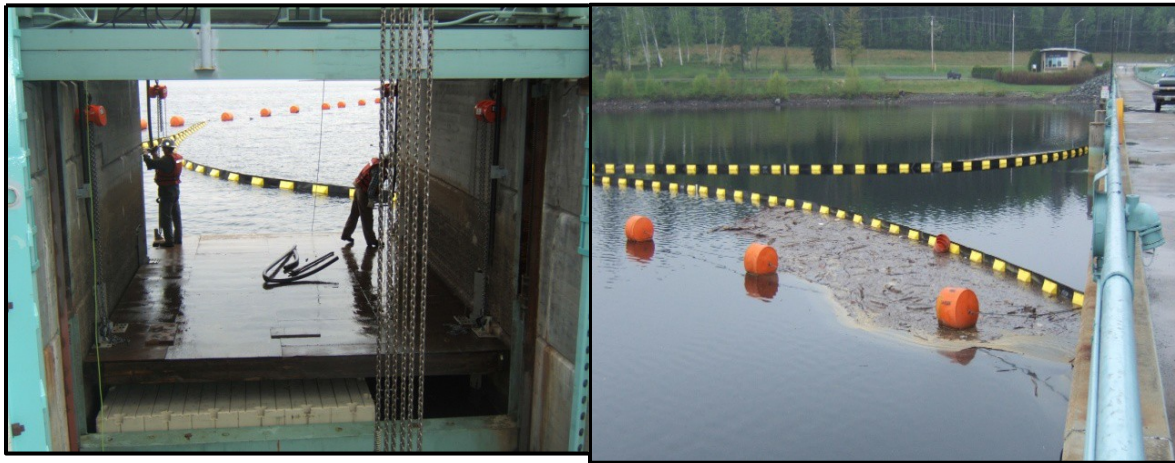
Figure 2-3. Moore fish sampler attraction flow shelf raised for repairs (left), view is looking upstream through the skimmer gate entrance to Moore Reservoir; and the debris boom (right).
