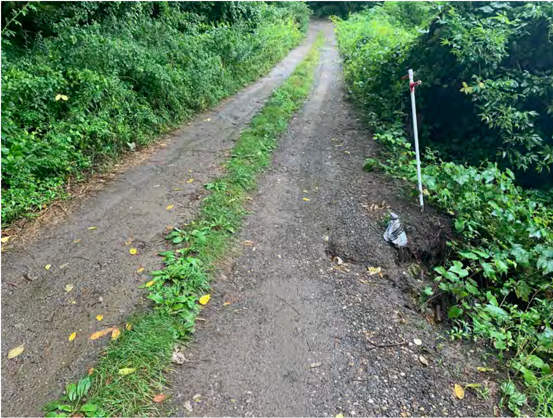
Photo 5: Eroded roadbed over culvert. Part of parcel 3
