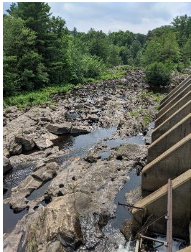
Figure 6b. Bypassed reach (upstream).
