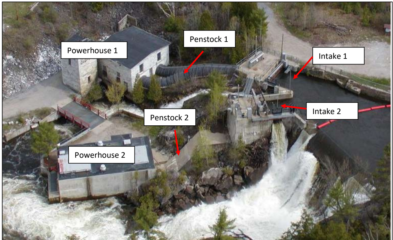
Photo B-4 – View of Beldens Intakes, Penstocks and Powerhouses
