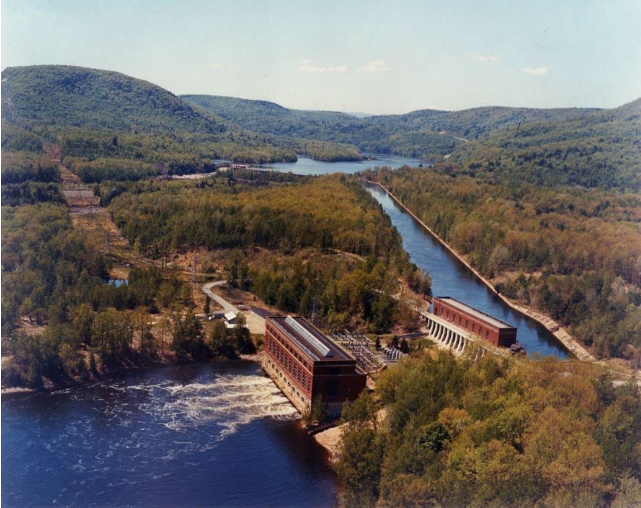
Figure 5 – Sherman Island Power Canal, Main Powerhouse, and Tailrace
