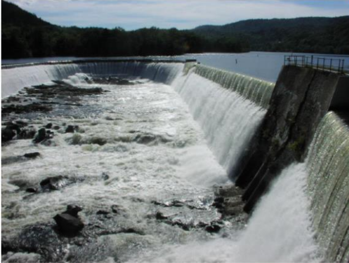
Figure 3 – Sherman Island Spillway
