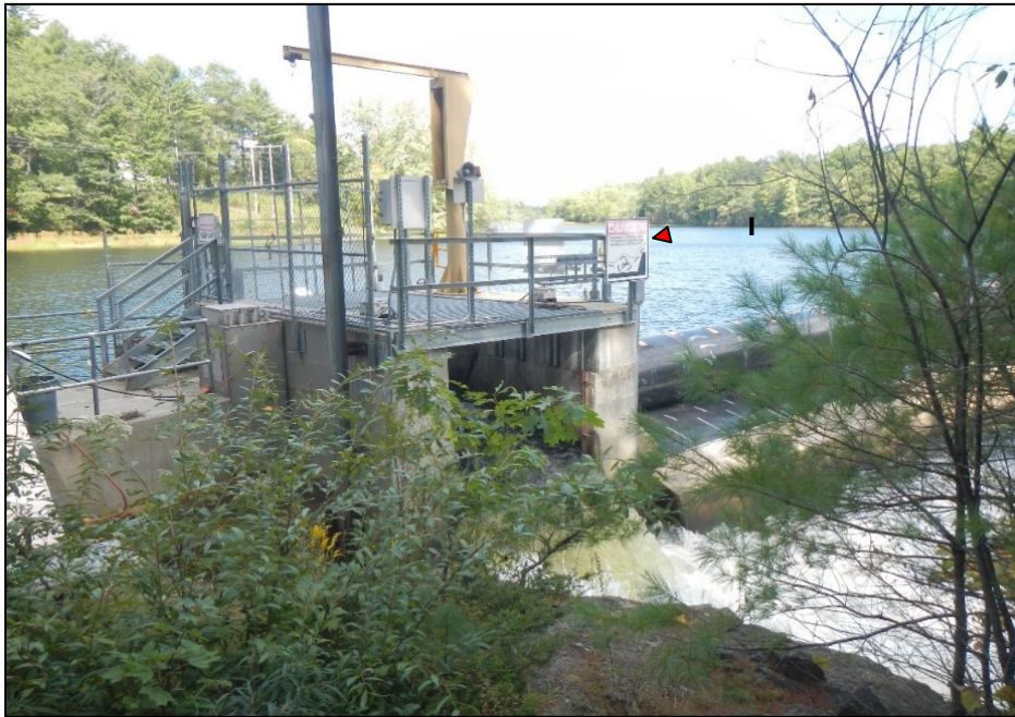
Figure 7 – Minimum Flow Gate at the Diversion Dam
