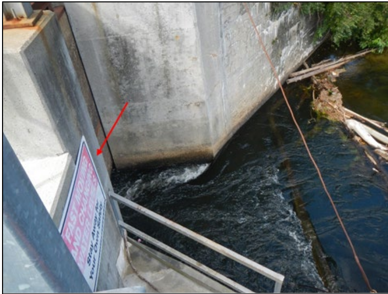
Figure 10 – Downstream Fish Passage Entrance
