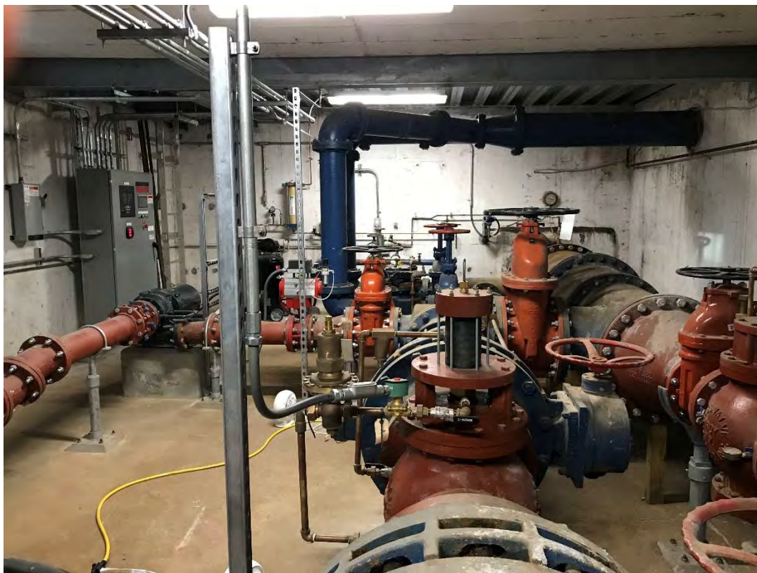
Photograph 2: Pumps and Hydroelectric generator located within facility.
