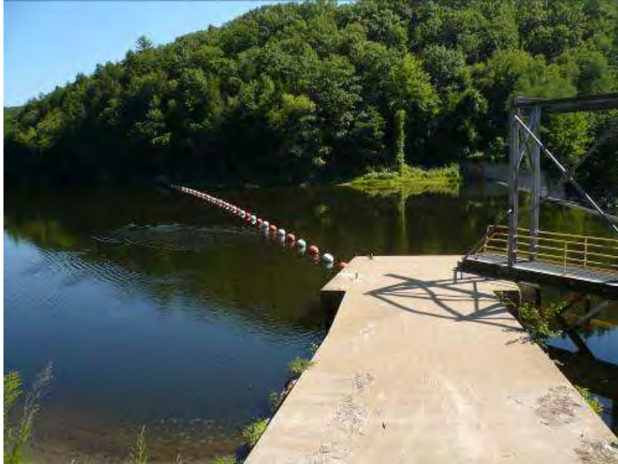
Photo 10: Boat barrier in place in project impoundment.
