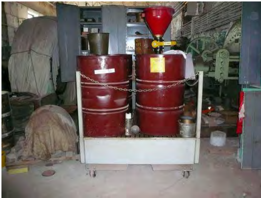
Photo 25: Secondary containment measures inside project powerhouse.
