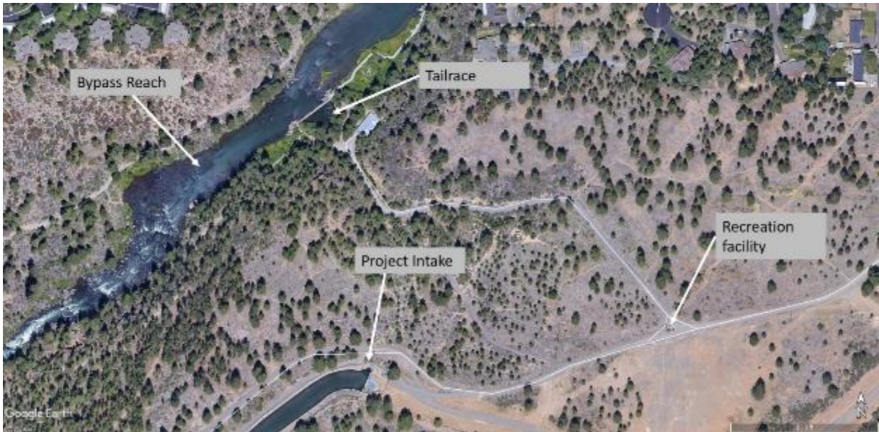
Figure 6 –Siphon Power Powerhouse Area.
