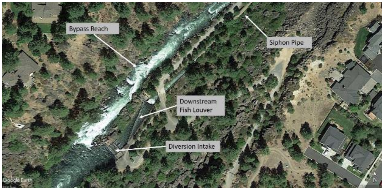
Figure 3 – Siphon Power Diversion Intake Area.
