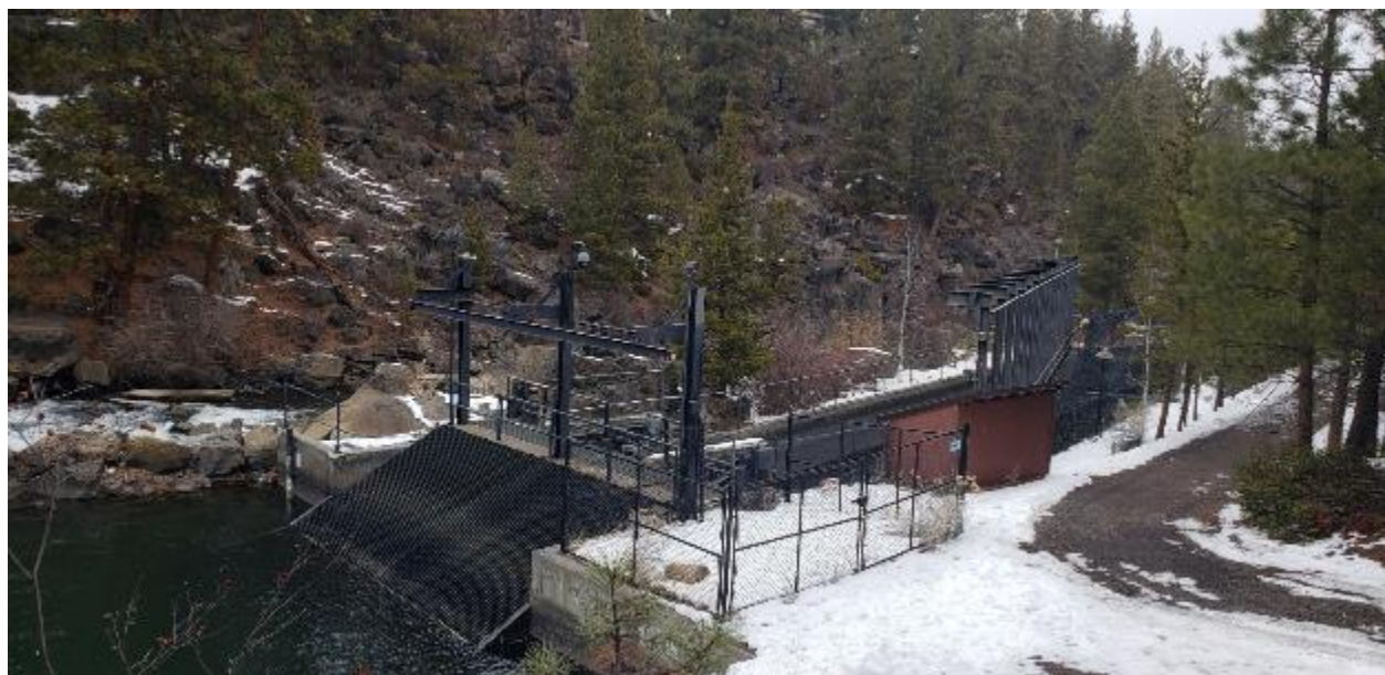
Figure 4 –Siphon Power Diversion Intake.
