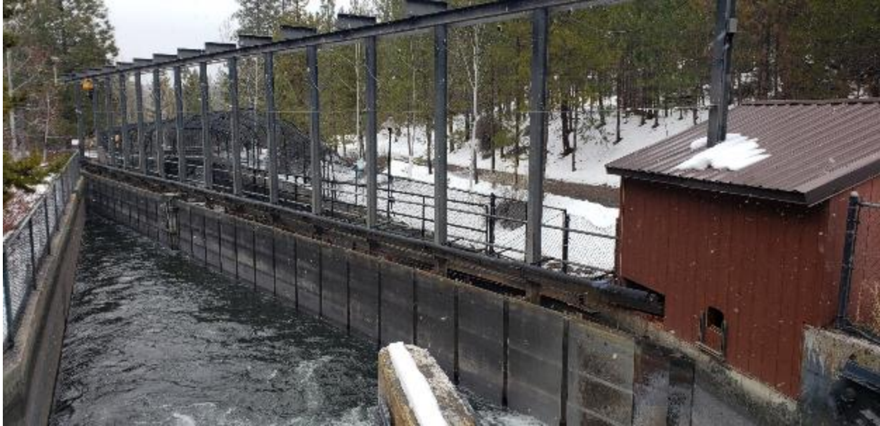
Figure 5 – Downstream Fish Louver Array.
