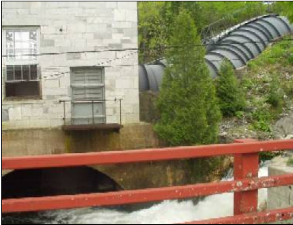
Photo 1-16 Beldens Steel Bifurcated Penstock Leading to Powerhouse-1
