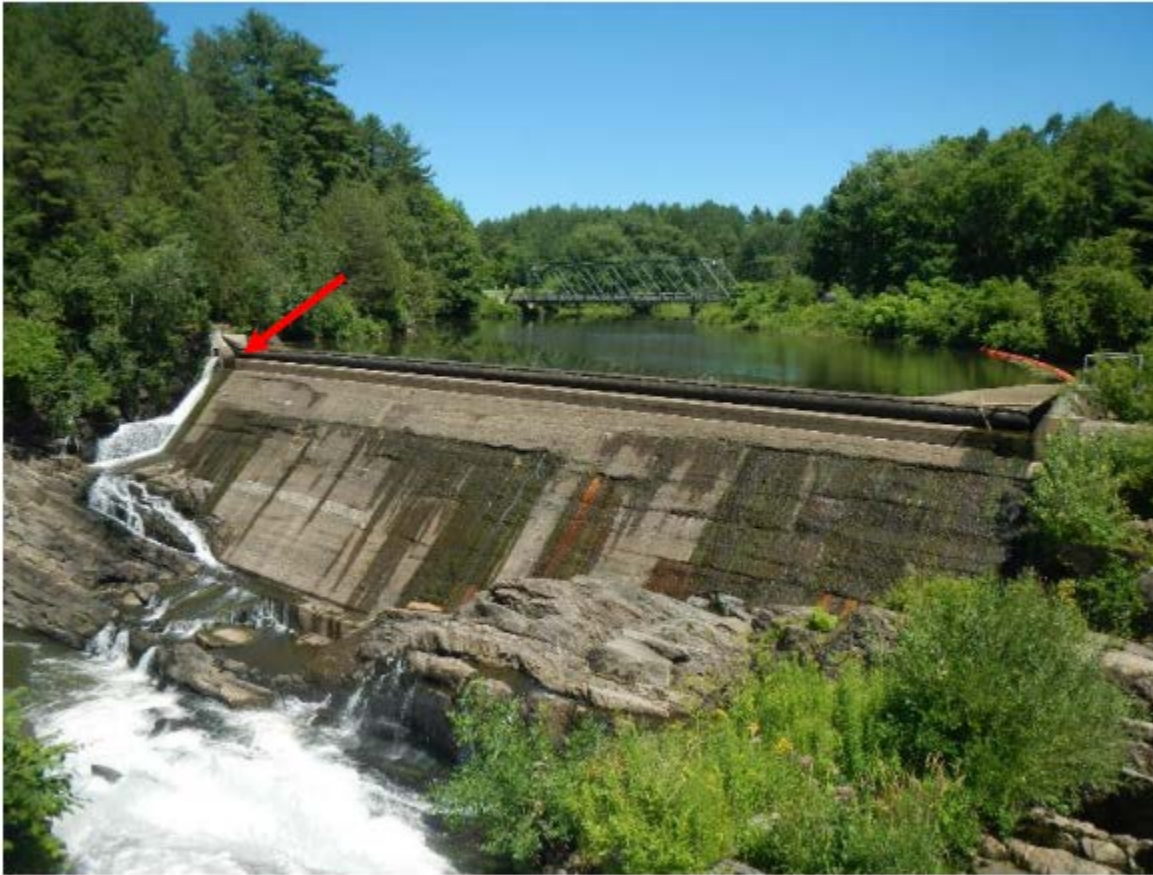
Photo 3-1 View of Minimum Flow Through the New Minimum Flow Gate on the Right Side of Huntington Dam
