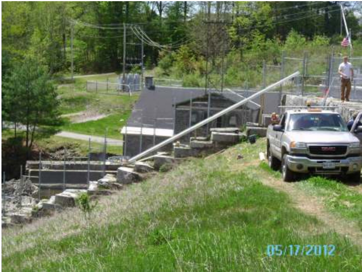
Top ramp temporarily set in place.
