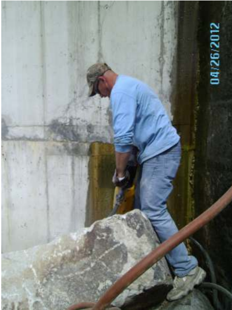
Breaking up of granite blocks.
