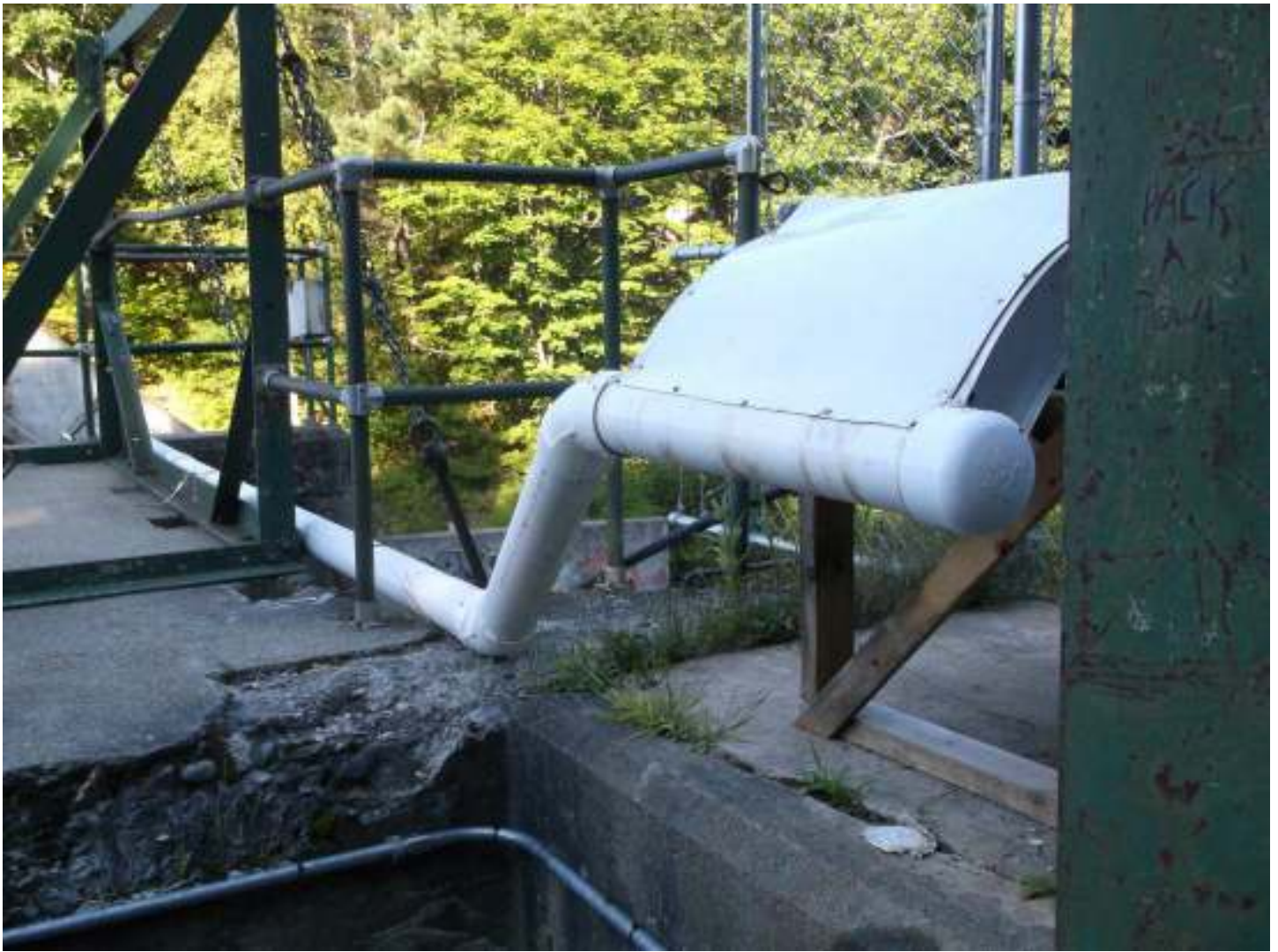
Piping across minimum flow gate
