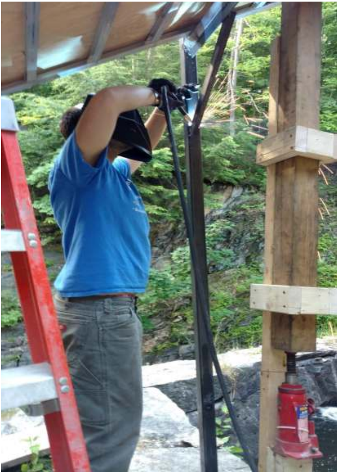
Permanent brackets being installed
