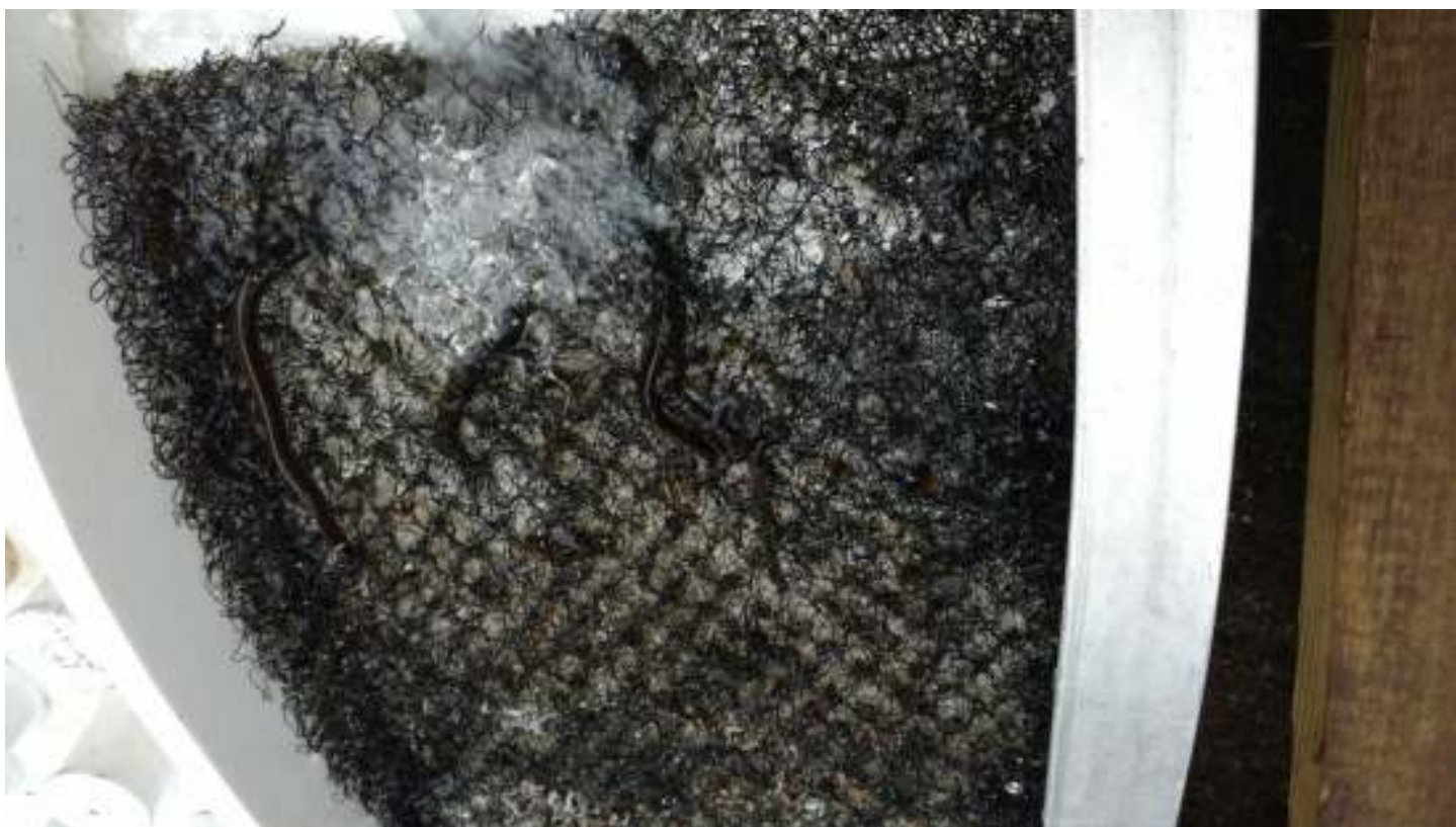
Eels climbing Enkamat side of terminal end
