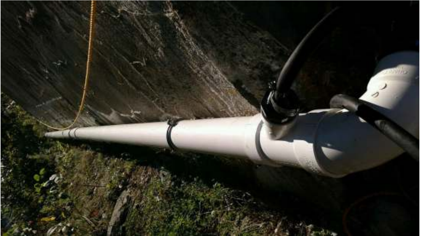
Exit pipe along Tower wall starting at terminal end with additional water supply
