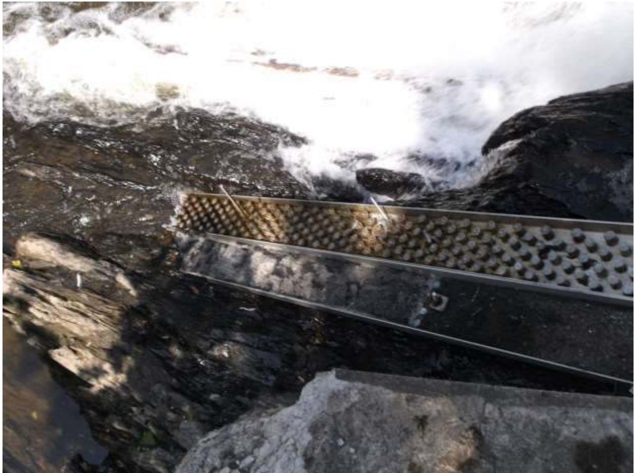
Entrance ramps reset with additional anchors
