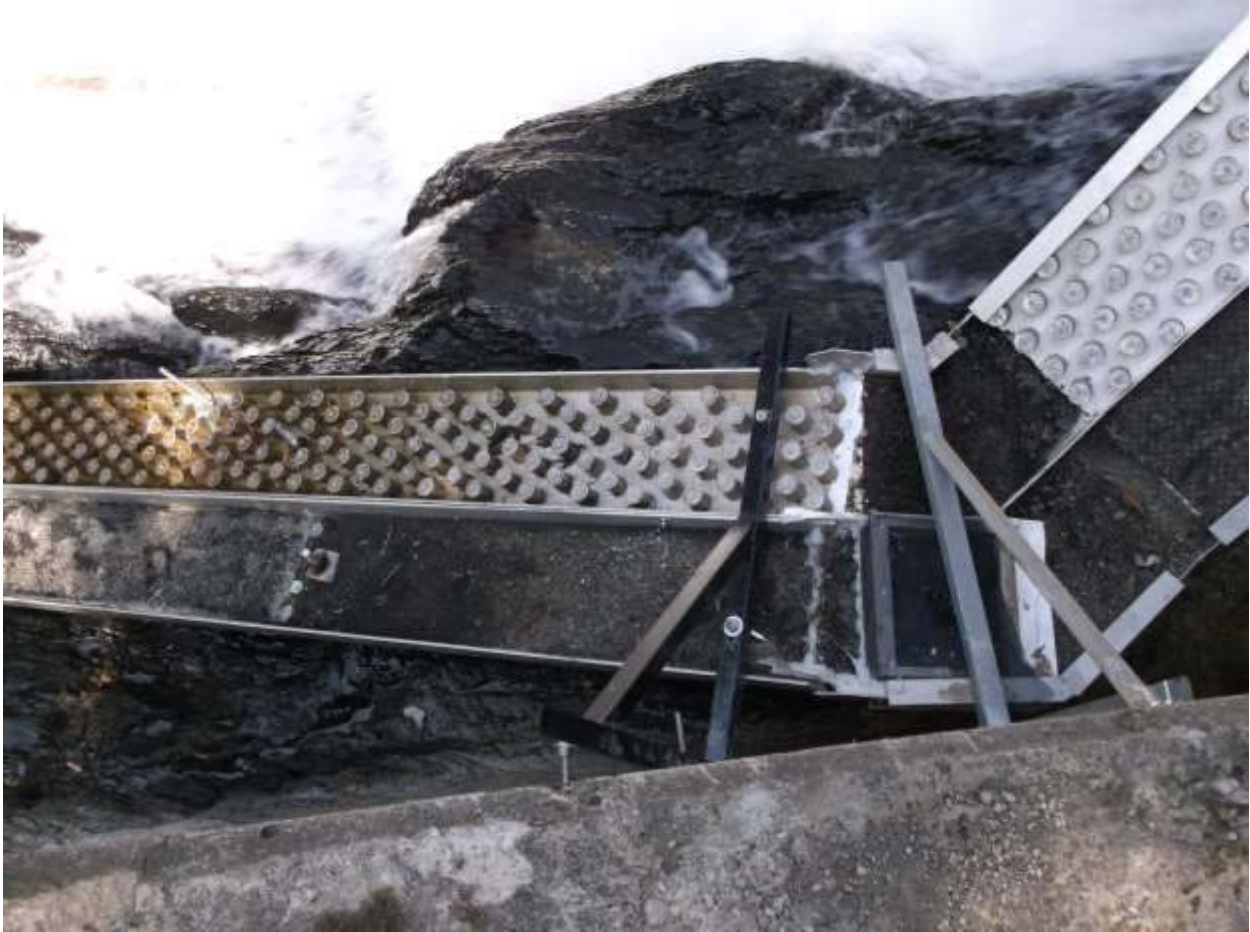
View of bracket and additional anchors
