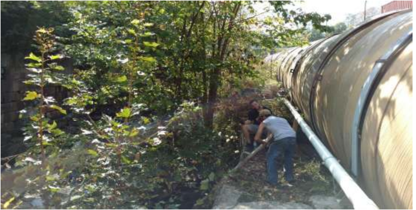
Pipe along penstock
