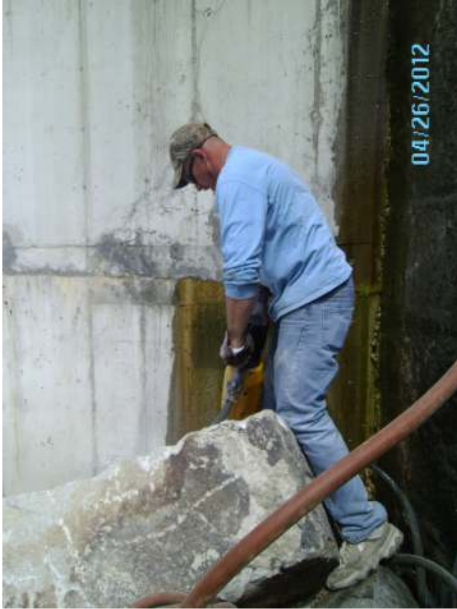
Breaking up of granite blocks.
