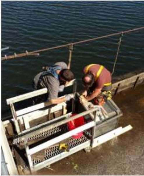
Left: Platform and eel trap installation Right: 1" coated screen installation on flashboard
