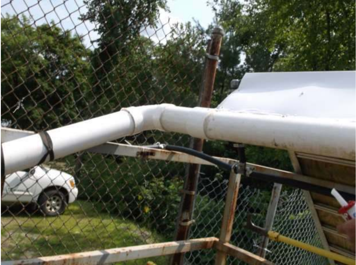
Permanent exit pipe and terminal end cover in place
