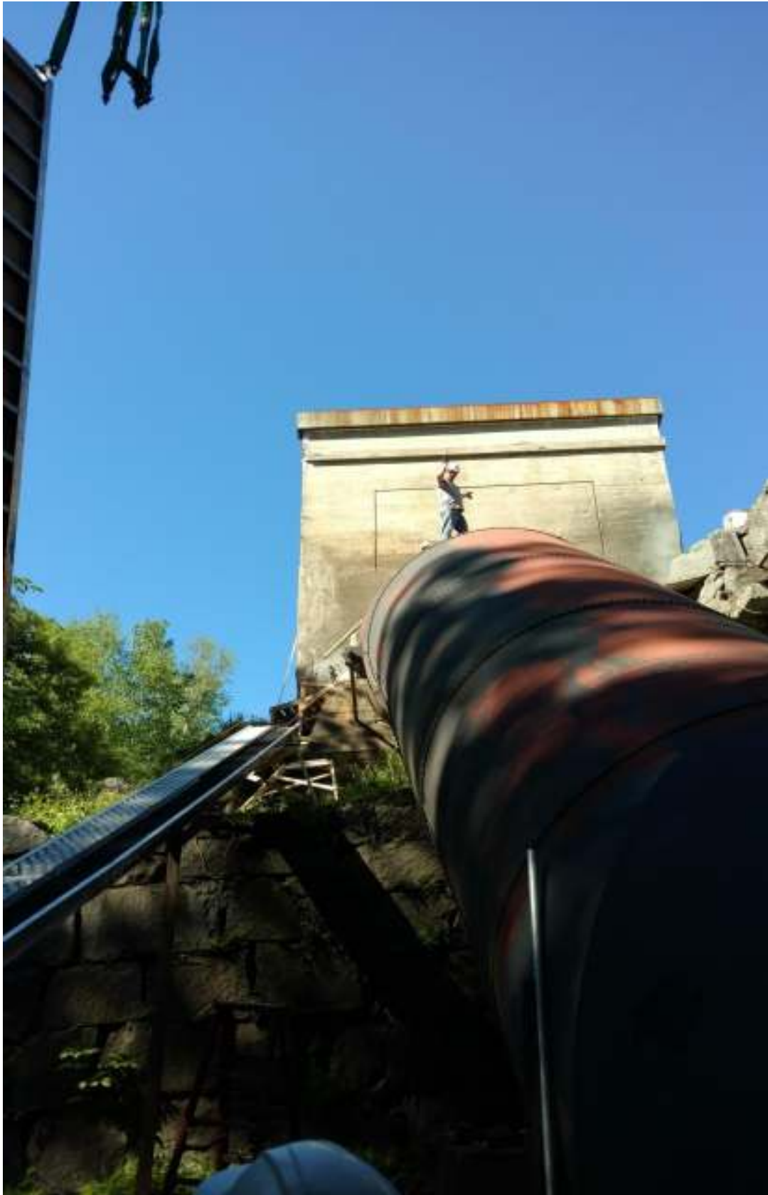
Top piece being lowered into position
