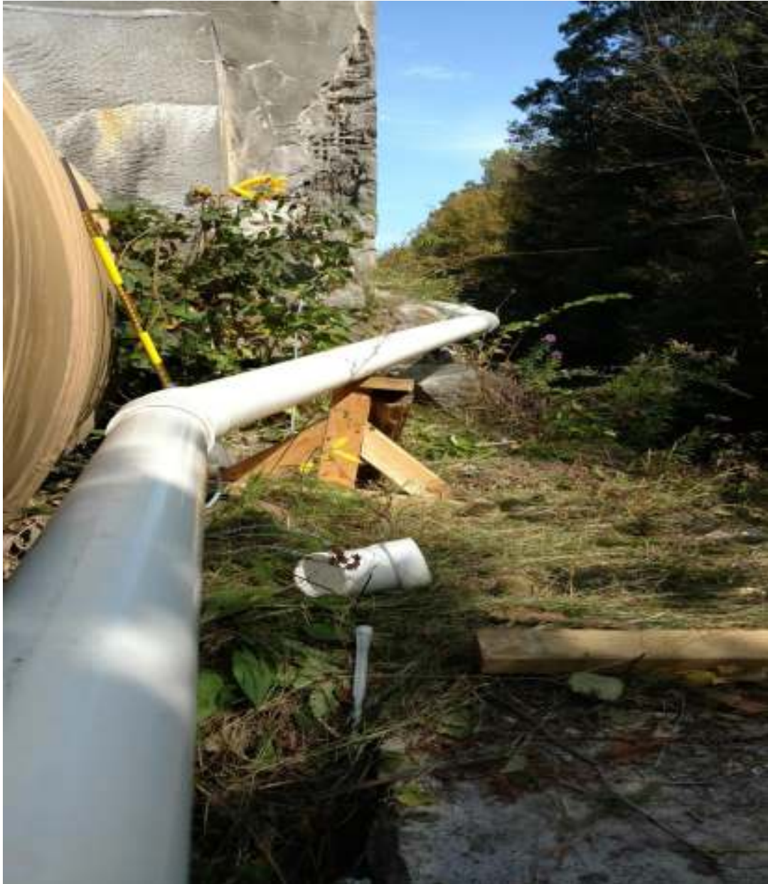
North side of tower showing exit pipe angled to penstock
