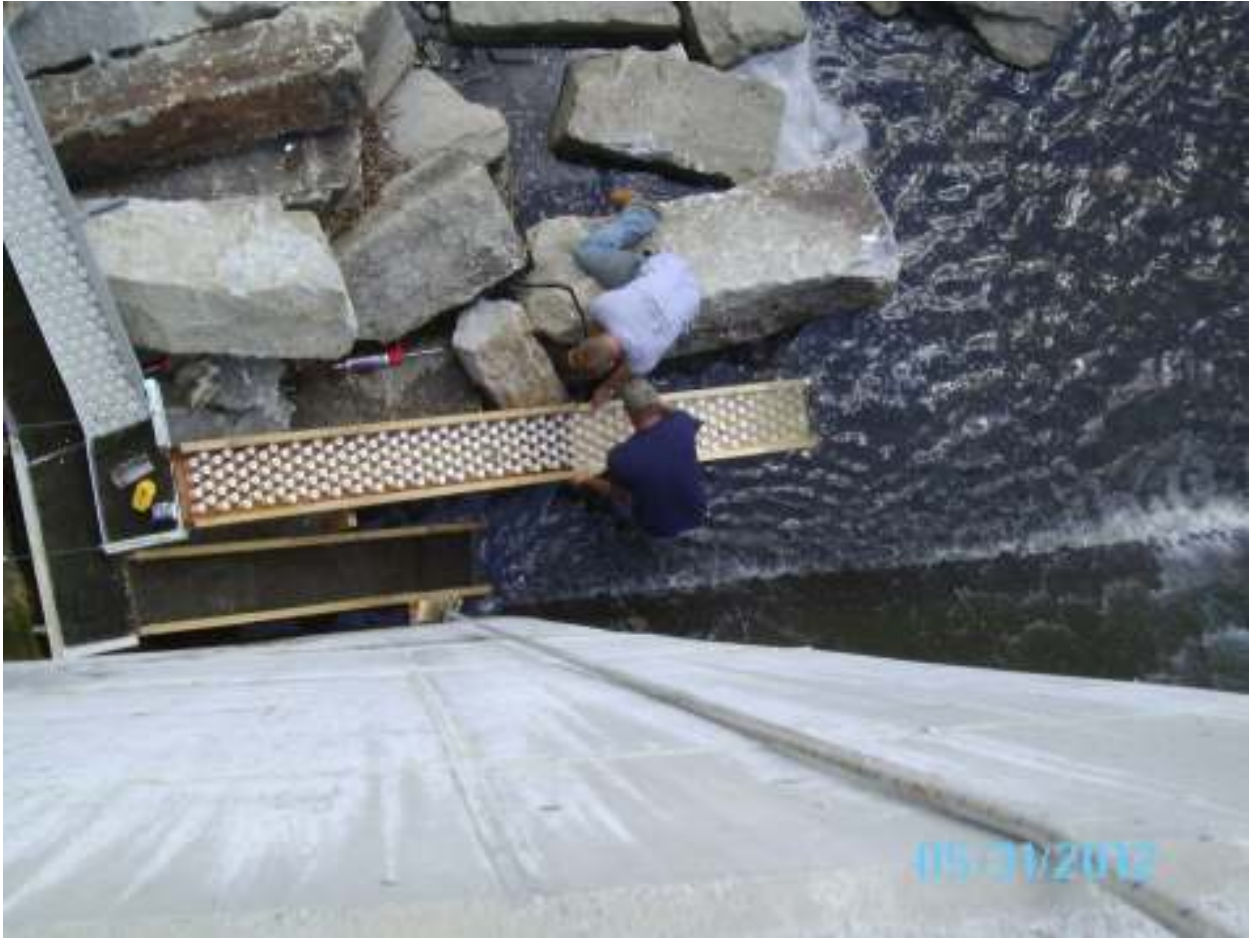
Final Ramp Assembly
