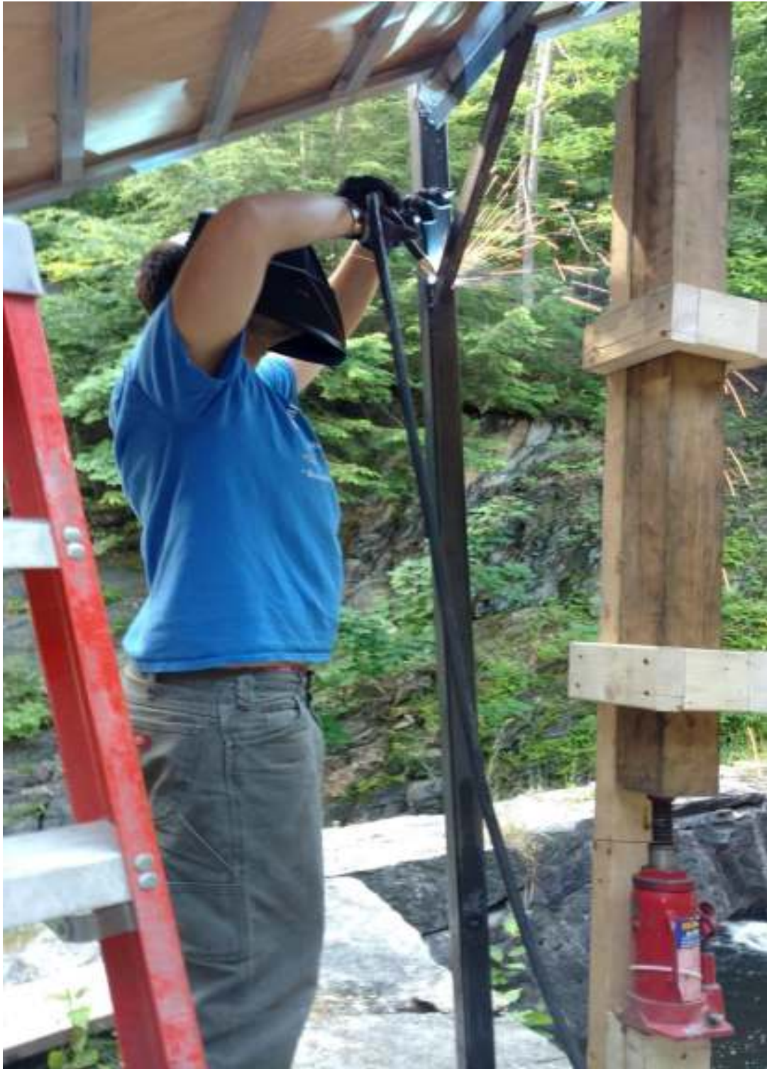
Permanent brackets being installed
