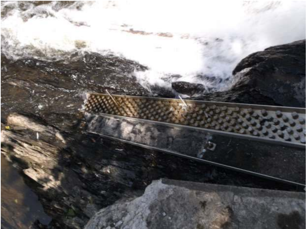
Entrance ramps reset with additional anchors
