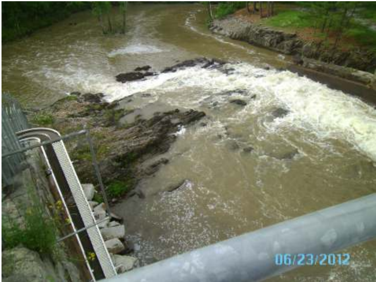
View from top of dam.
