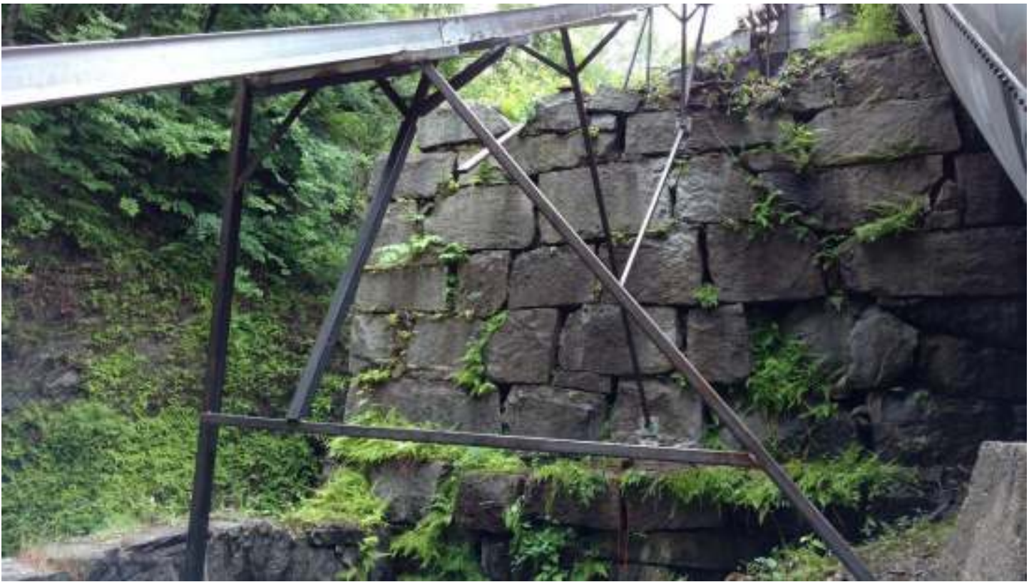
View of brackets and bracing
