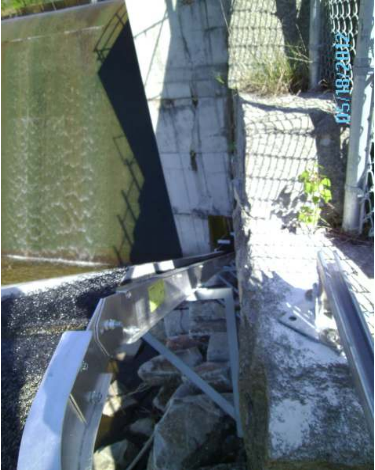
Transition pool bolted to lower ramp assembly.
