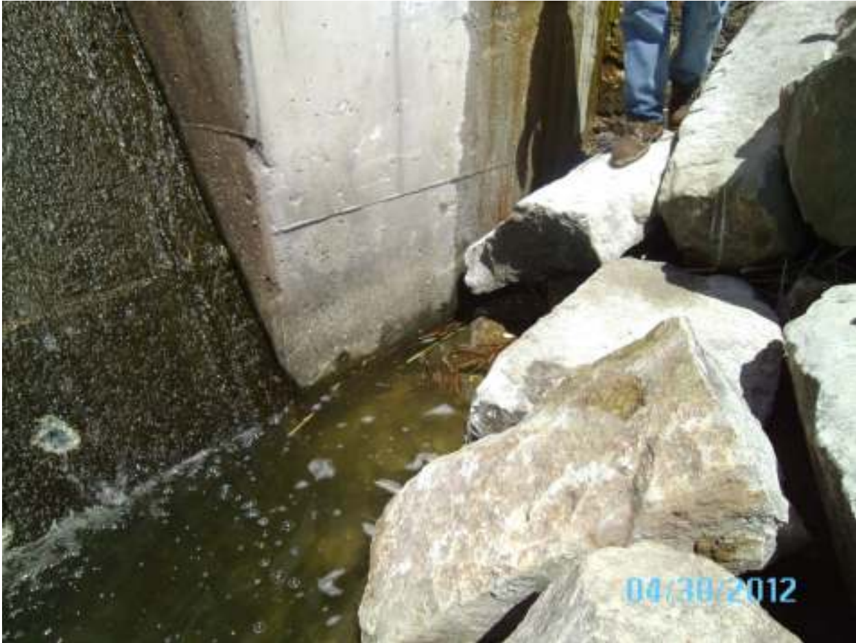
Corner after granite removal.
