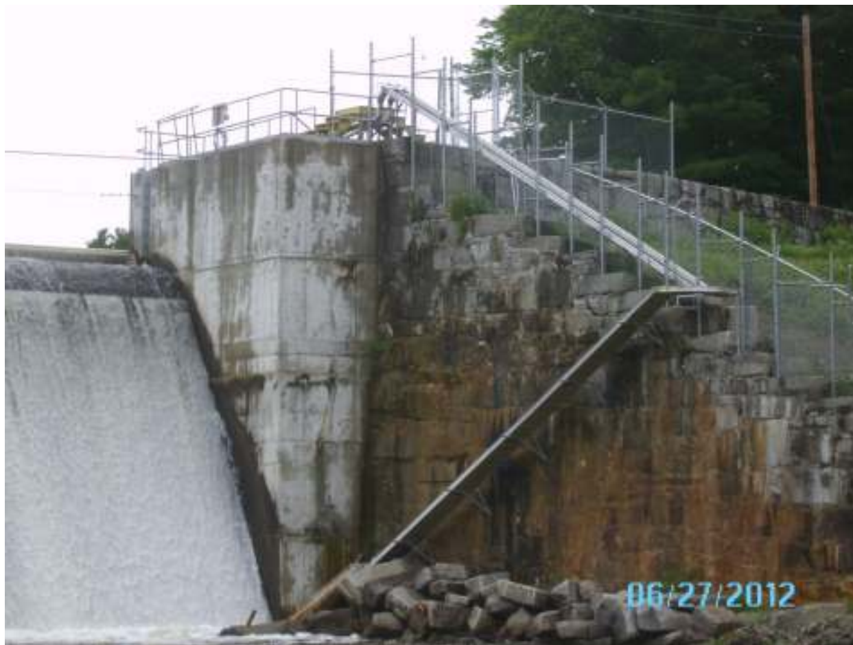
Completed Eel Passage
