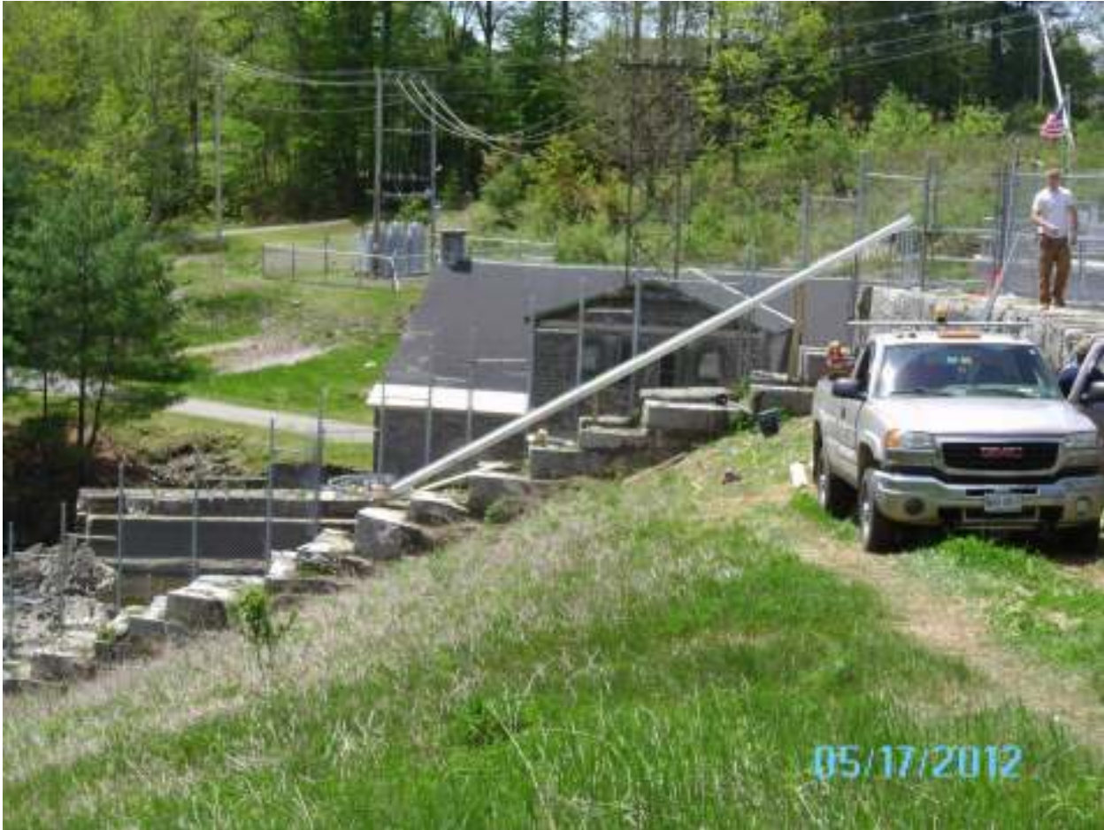
Top ramp temporarily set in place.
