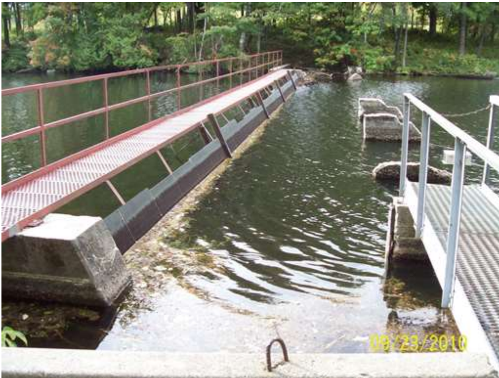
Messalonskee Lake Dam (Snow Pond) fish rack upstream side.
