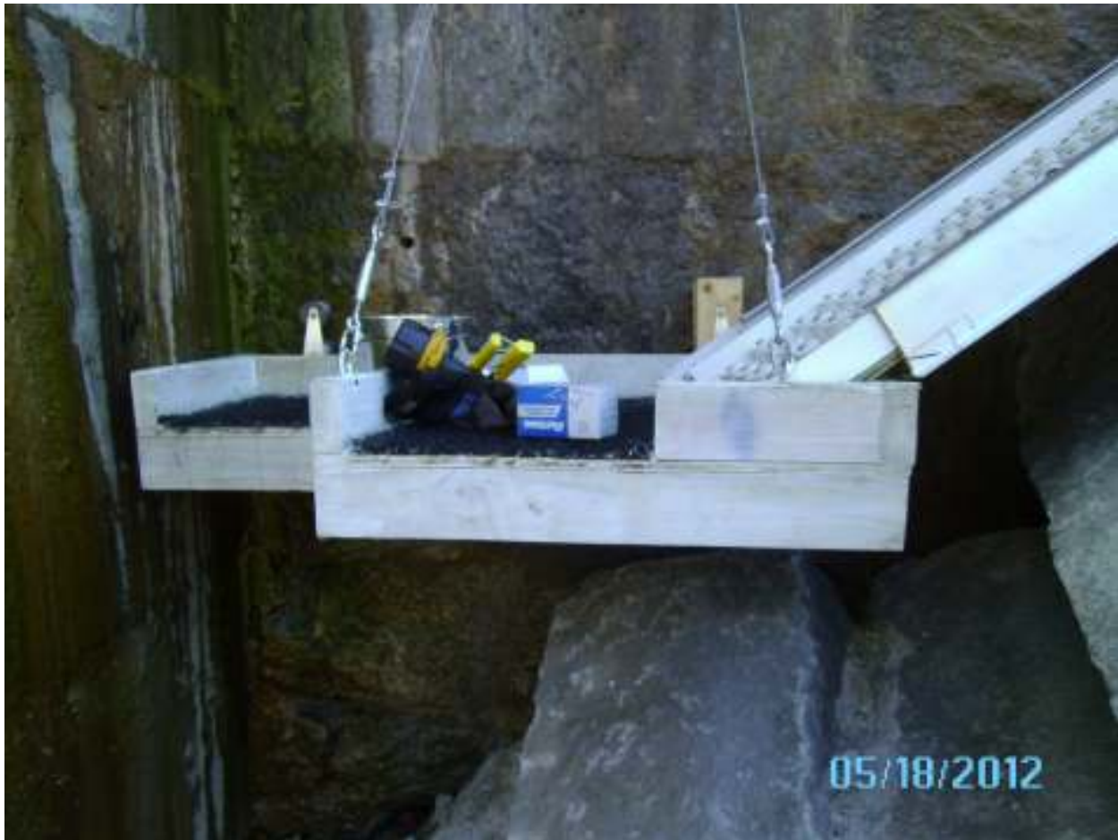
Corner pool installed
