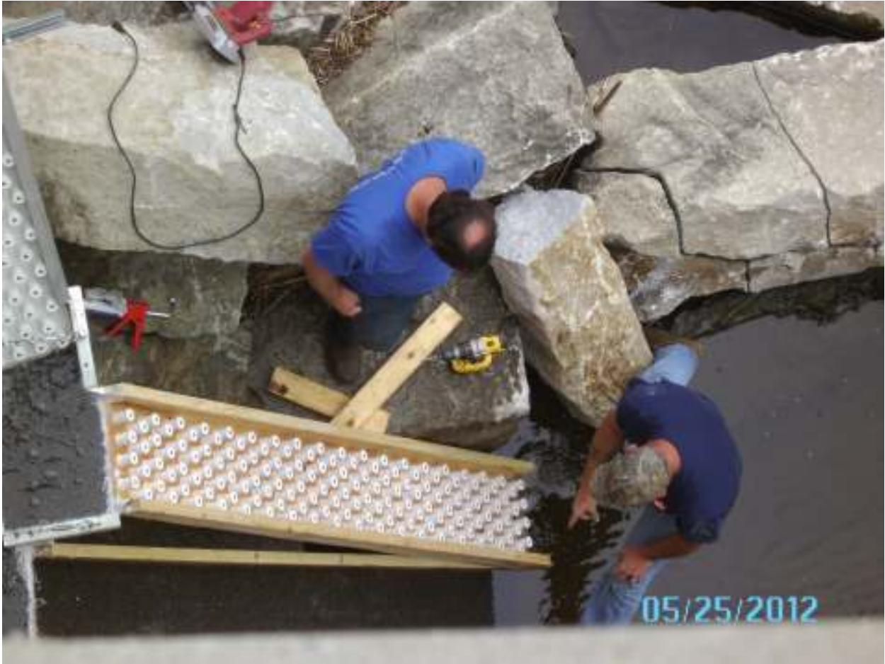
Original Ramp installation
