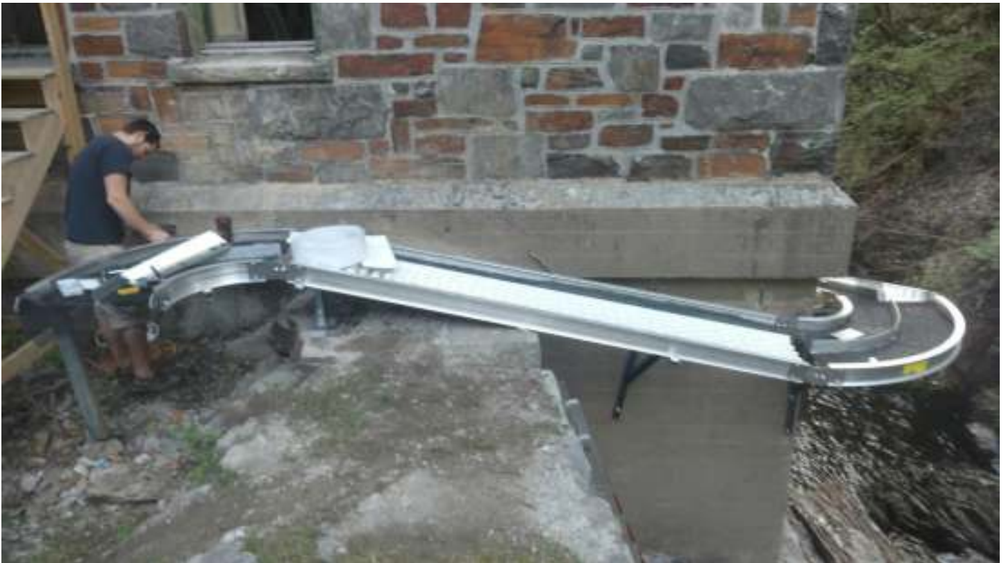
North side generation building
