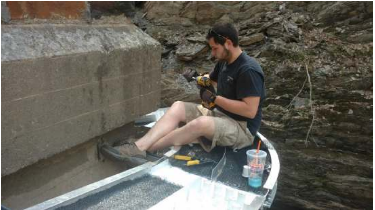
90° section on northwest corner being attached
