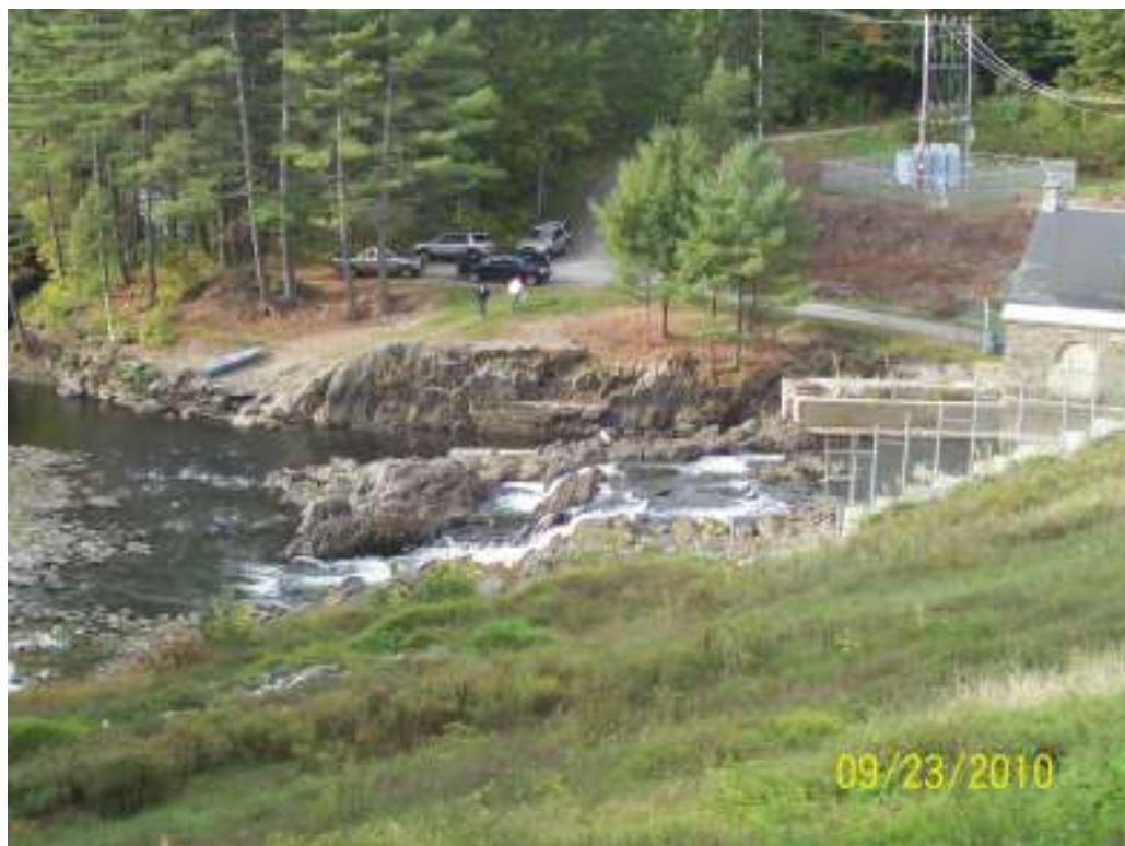
Ledges below spillway from river left
