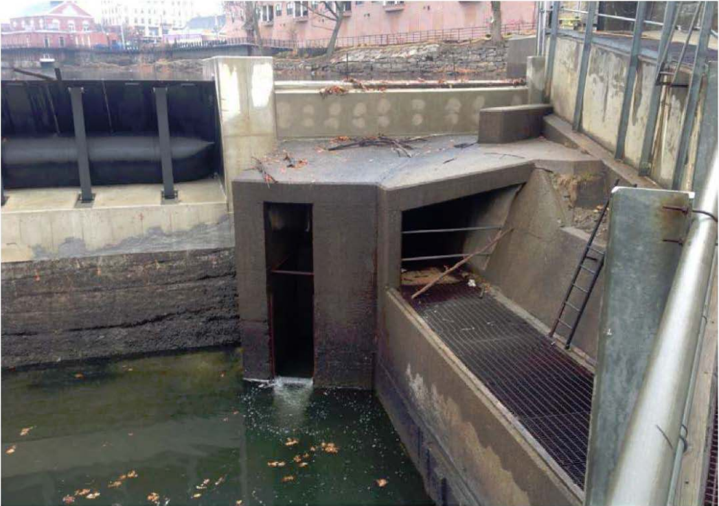
Figure 3. Spillway channel and top of fish ladder
