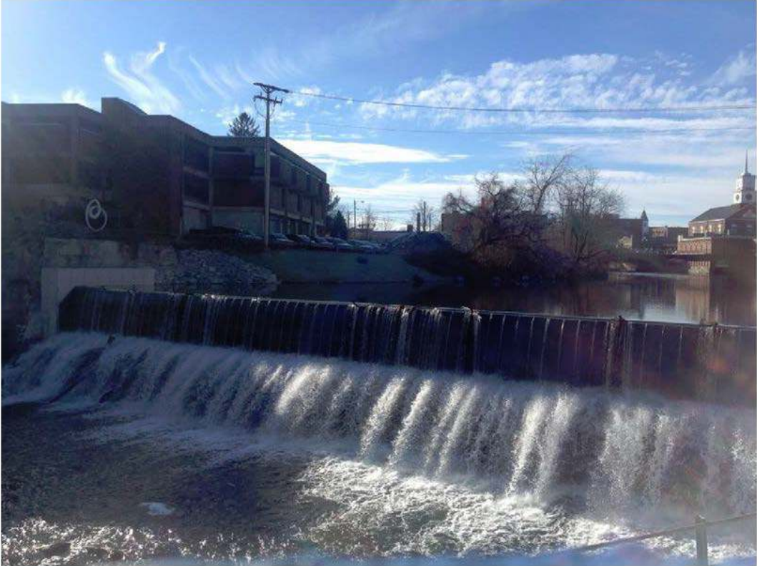
Figure 2. Dam and pneumatic crest gates
