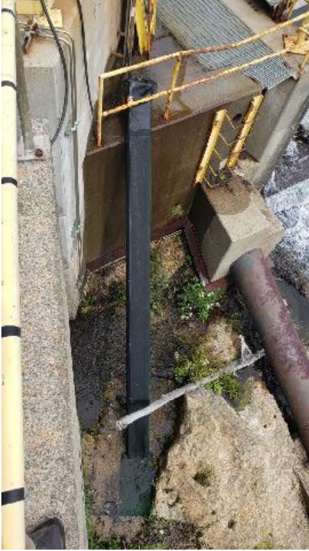
Figure 7 – Upstream Eel Passage System
