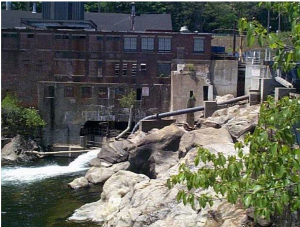
Figure 6 –Powerhouse with Downstream Fish Bypass in Foreground
