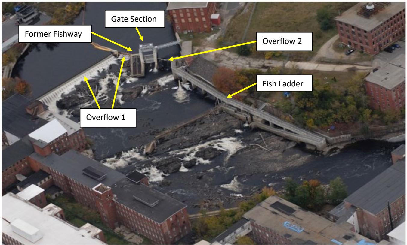
Figure 5 - West Channel Dam
