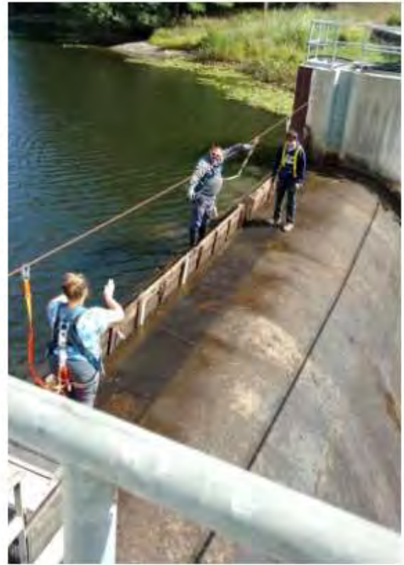
Left: Platform and eel trap installation Right: 1" coated screen installation on flashboard
