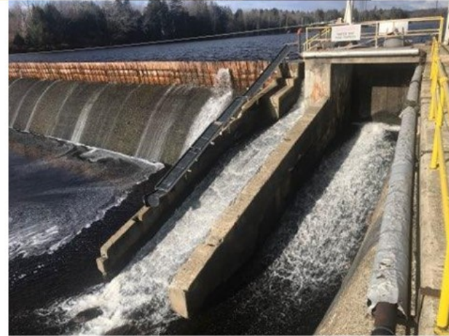
M3: DS Bypass Sluice
