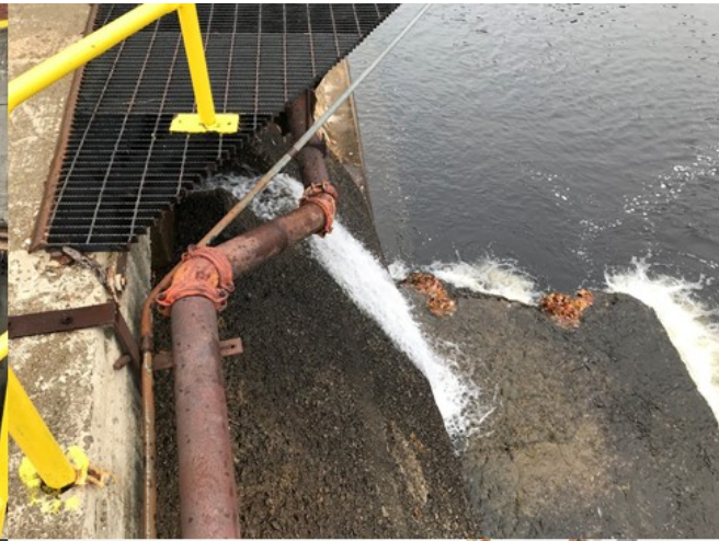
M4: Forebay Sluice
