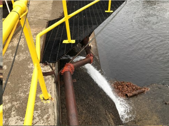
M4: Forebay Sluice
