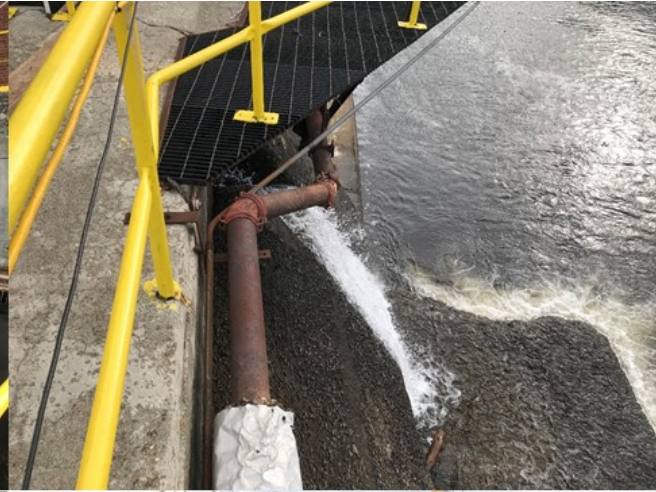
M4: Forebay Sluice
