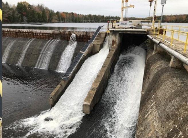
M3: DS Bypass Sluice
