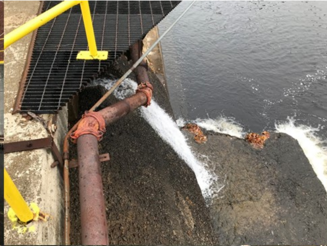
M4: Forebay Sluice
