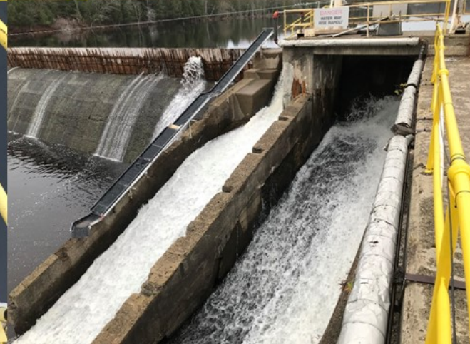
M3: DS Bypass Sluice
