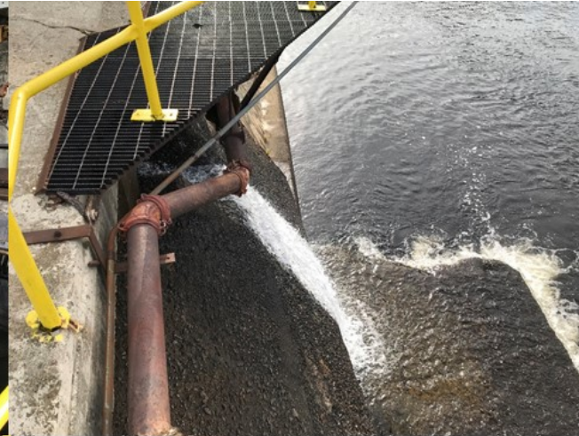
M4: Forebay Sluice
