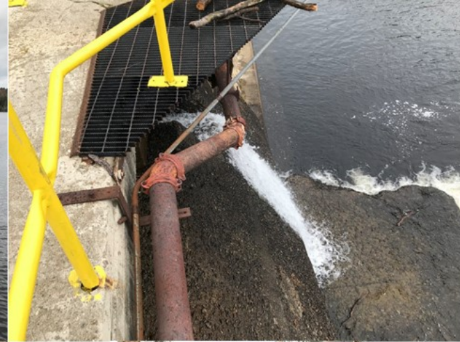
M4: Forebay Sluice
