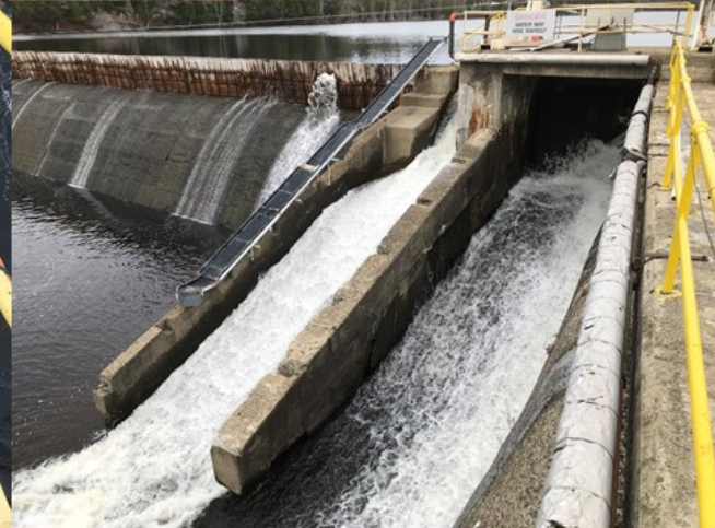
M3: DS Bypass Sluice
