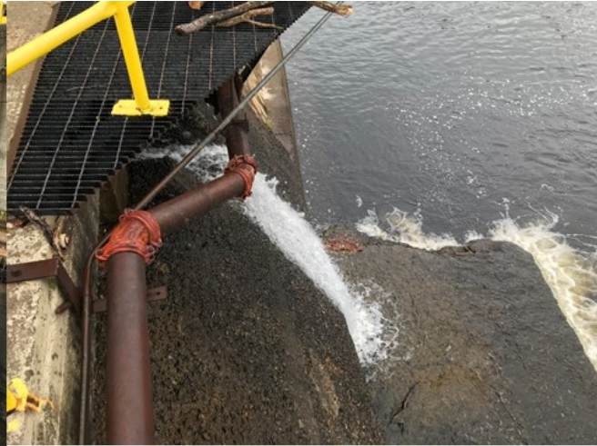
M4: Forebay Sluice
