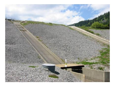
The dam is an earth and rock zone fill approximately 1350 feet long with a top width of 28 feet. Height of the dam is 106 feet and water depth at the spillway crest elevation is 100 feet. Construction was under the authority of the Watershed Protection and Flood Prevention Act (Public Law 566).
