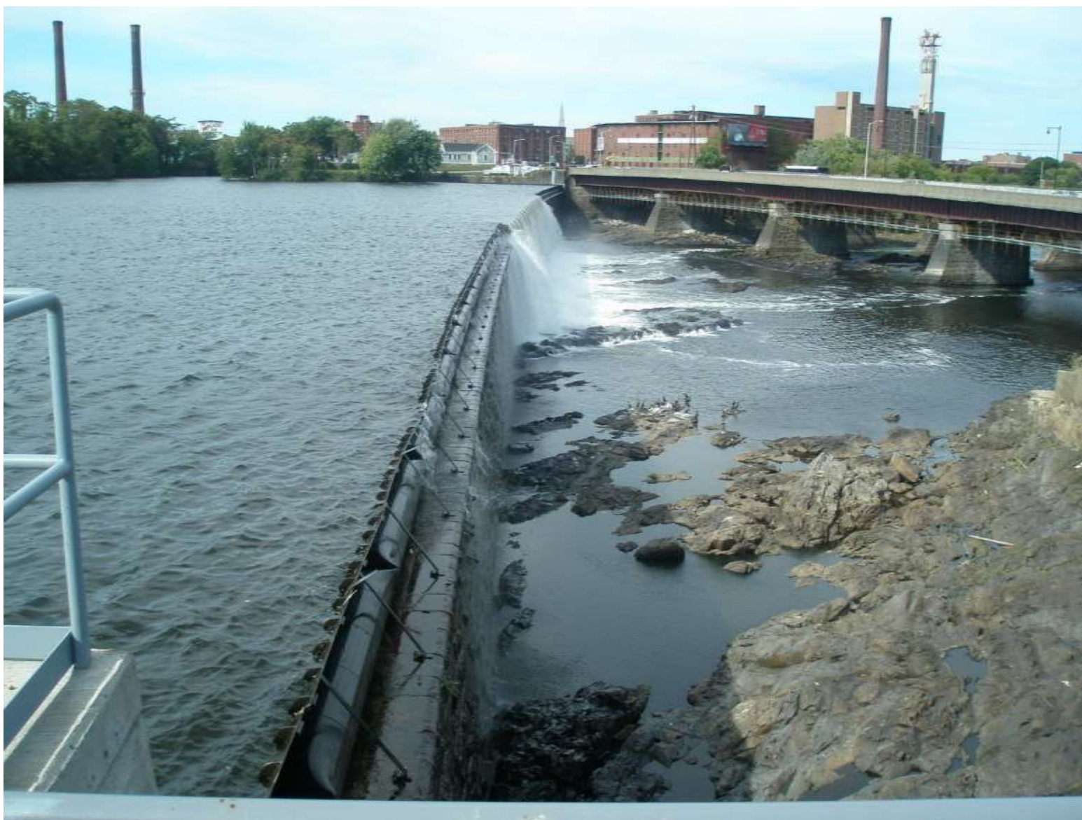
FIGURE 5: Lawrence Project impoundment, Essex Dam with the five-foot-high pneumatic crest gate system, the impoundment and downstream reach, and the North Canal Gatehouse in the background.
