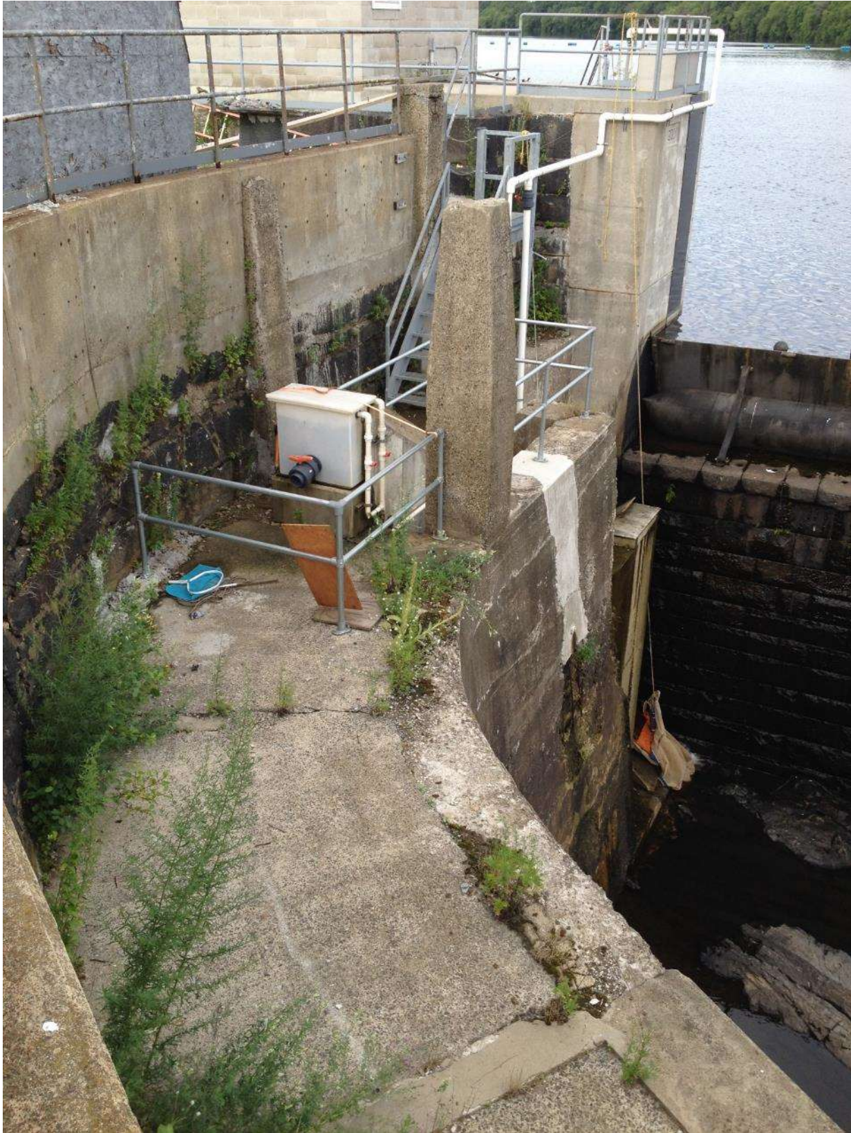
FIGURE 7: View of the eel collection tank that is part of the upstream eel passage system at the Lawrence Project.
