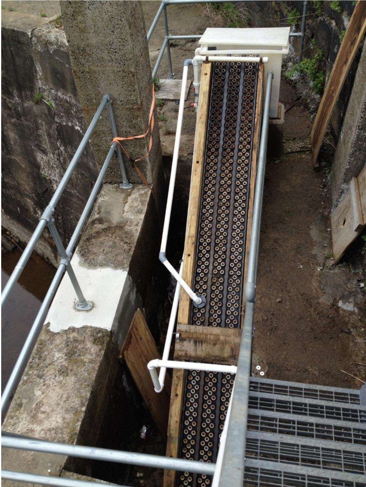
FIGURE 8: View of the upstream eel ladder at the Lawrence Project.
