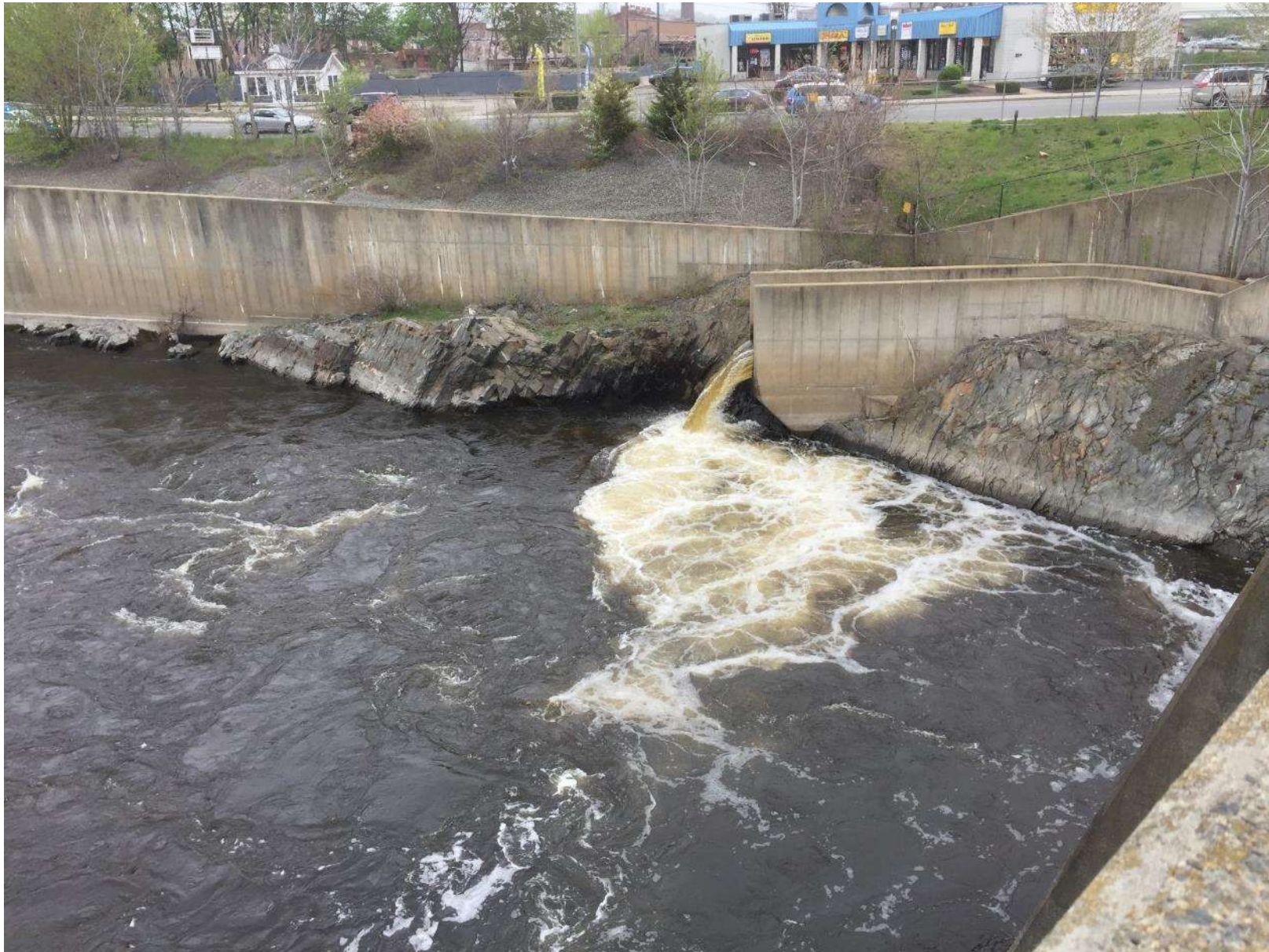
FIGURE 6: Lawrence Project tailrace and exit channel of the downstream fish passage facility.
