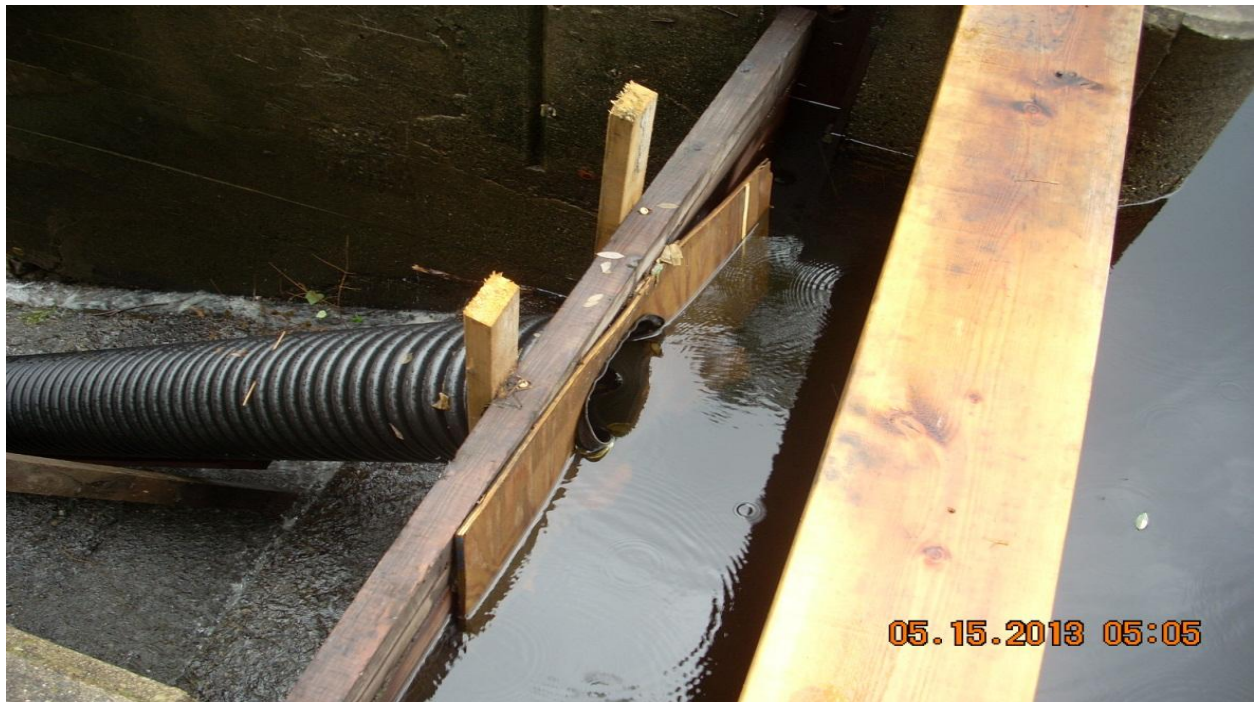
Temporary downstream eel passage installed at existing powerhouse while permanent downstream passage was being installed.
