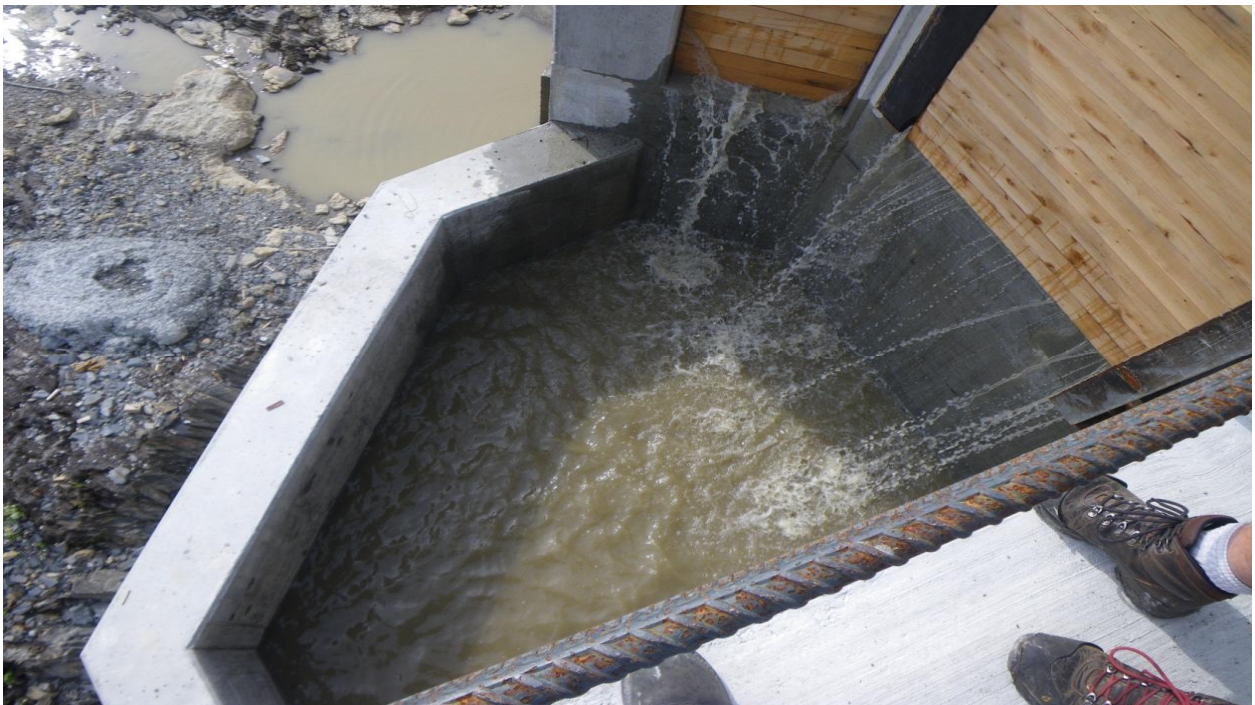
Plunge pool below eel and fish weirs.
