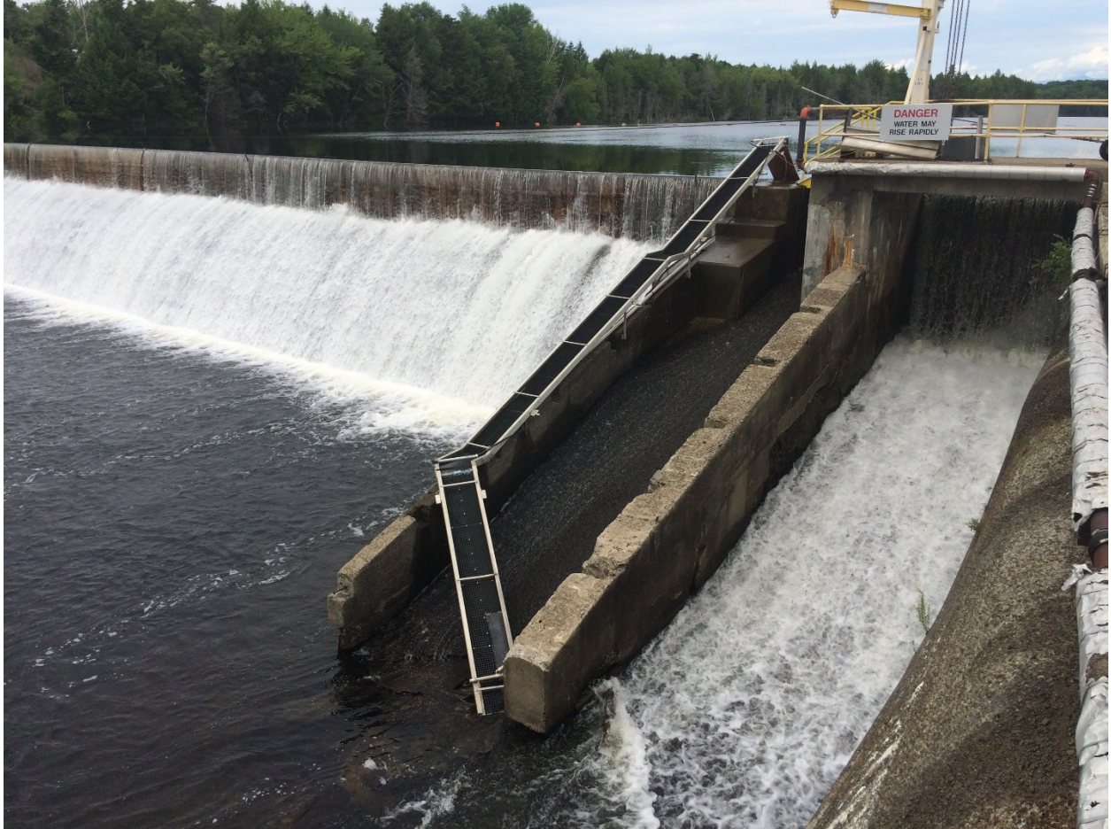
FIGURE 3. PROJECT FACILITIES – MEDWAY PROJECT (SPILLWAY AND EEL LADDER)
