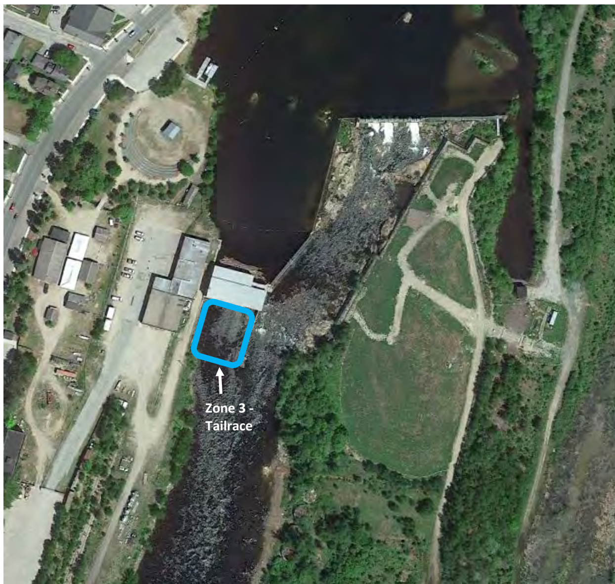
FIGURE 2-3 SAWMILL PROJECT – ZONE 3 - TAILRACE
