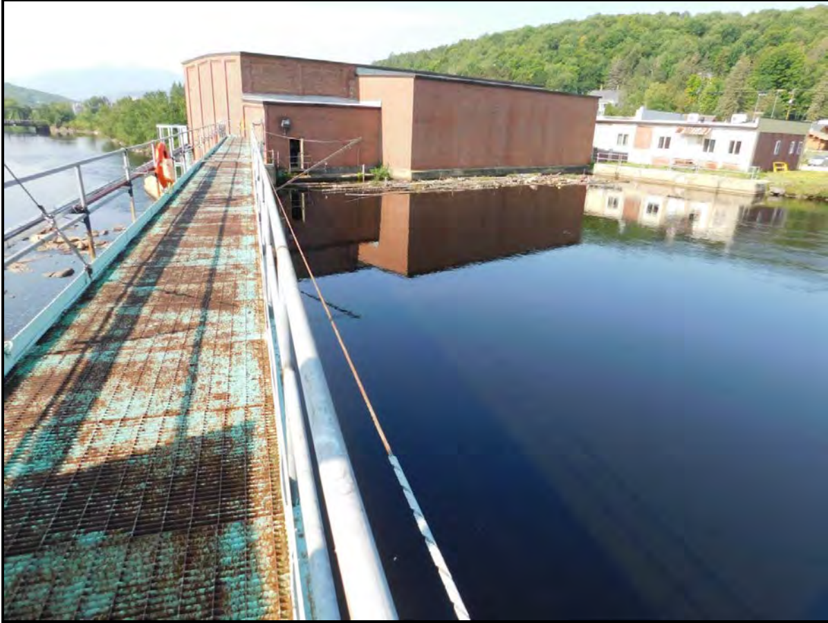
PHOTO 1-2 VIEW OF THE SAWMILL PROJECT GATEHOUSE AND POWERHOUSE.
