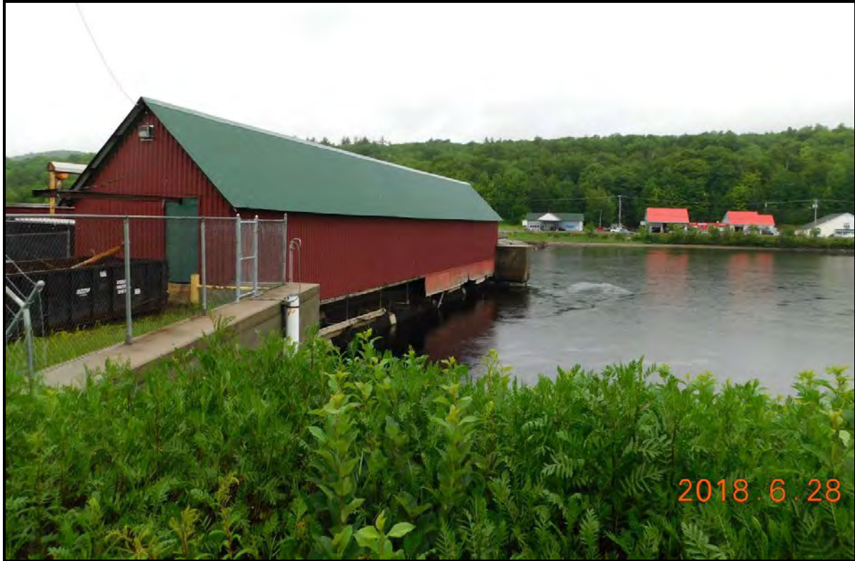
PHOTO 1-4 VIEW OF THE CROSS POWER PROJECT GATEHOUSE.
