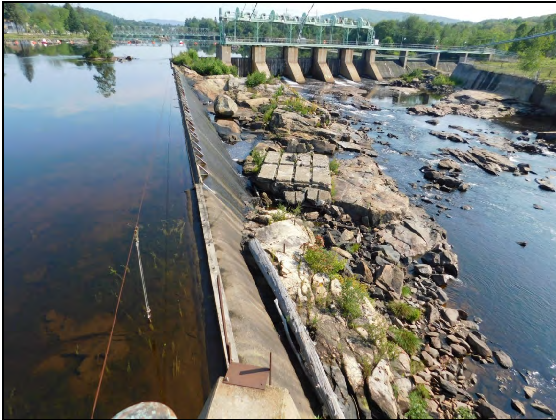
PHOTO 1-1 VIEW OF THE SAWMILL PROJECT DAM, WASTEGATES, SPILLWAY, AND BYPASSED REACH.
