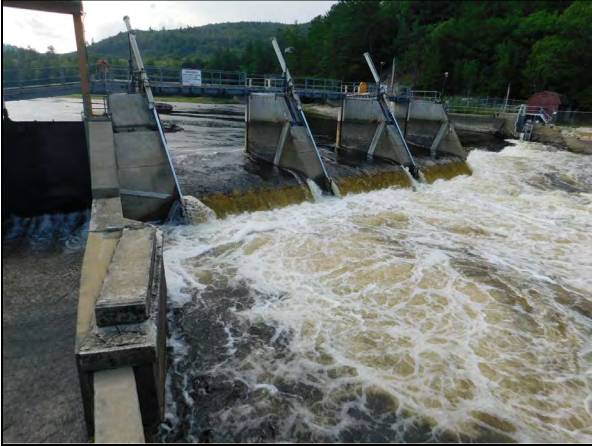
PHOTO 1-10 DOWNSTREAM VIEW OF SHELburne PROJECT SLUICEWAY, WASTEGATES, AND SPILLWAY
