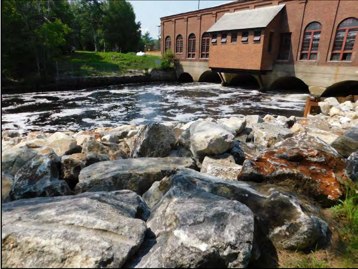
PHOTO 1-8 VIEW OF UPPER GORHAM PROJECT POWERHOUSE AND TAILWATER.
