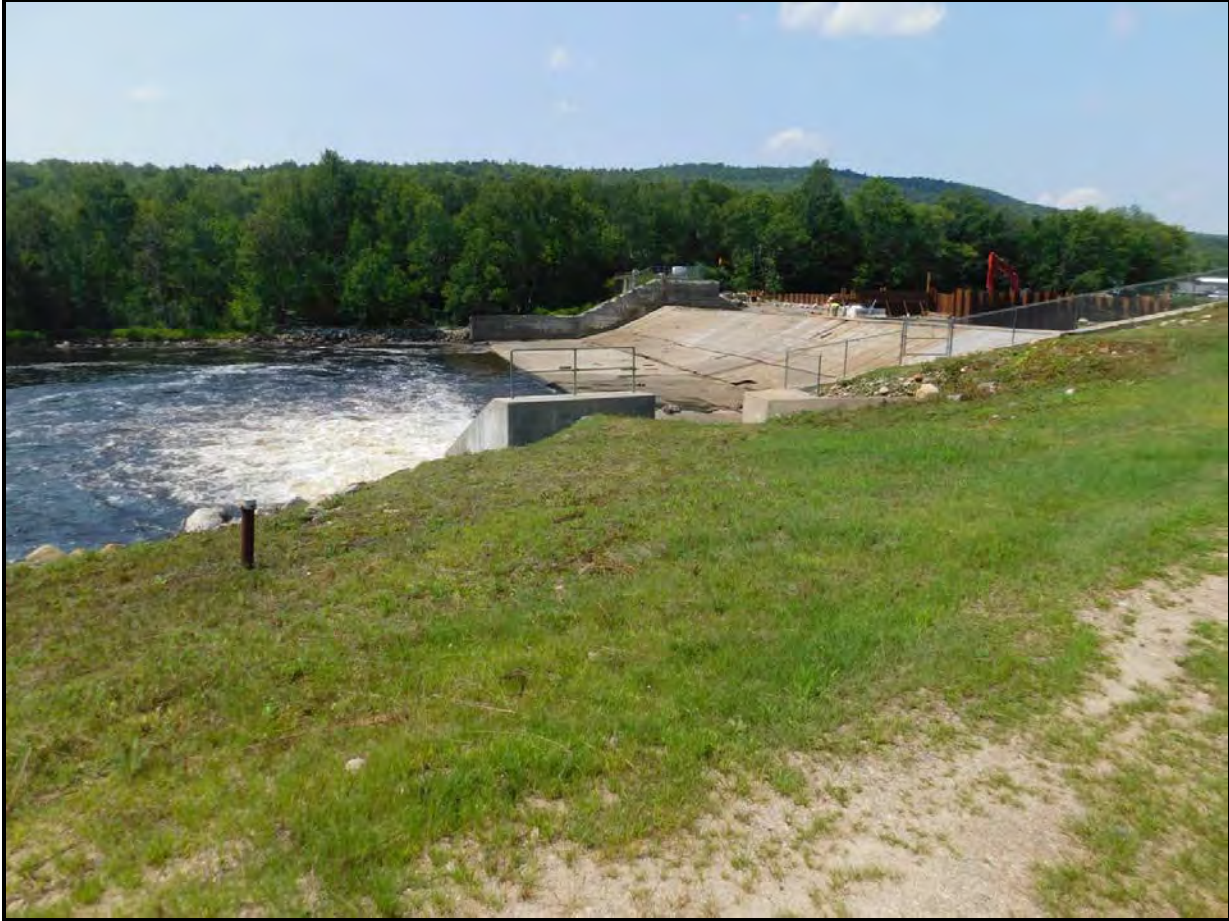
PHOTO 1-6 VIEW OF UPPER GORHAM DAM AND MINIMUM FLOW STRUCTURE.
