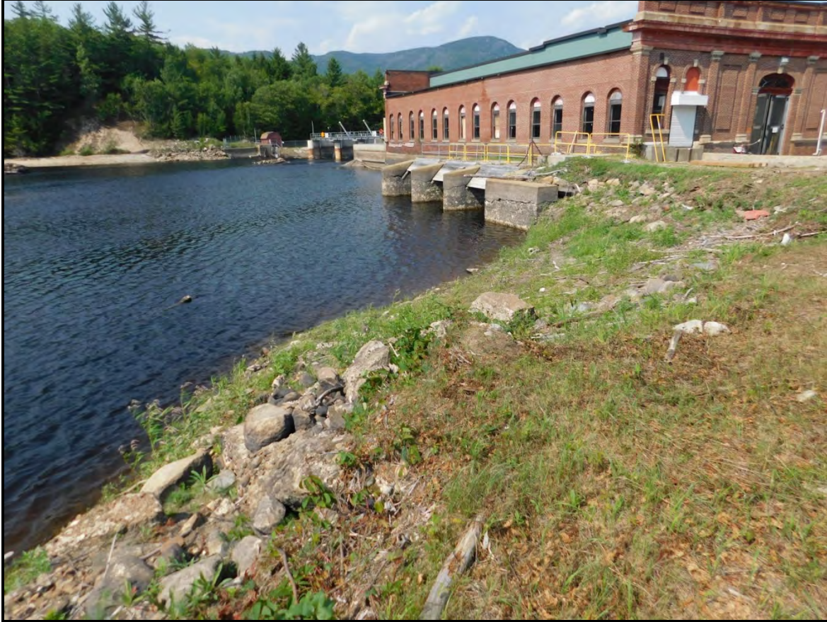
PHOTO 1-11 VIEW OF SHELBURNE PROJECT POWERHOUSE AND HEADPOND.
