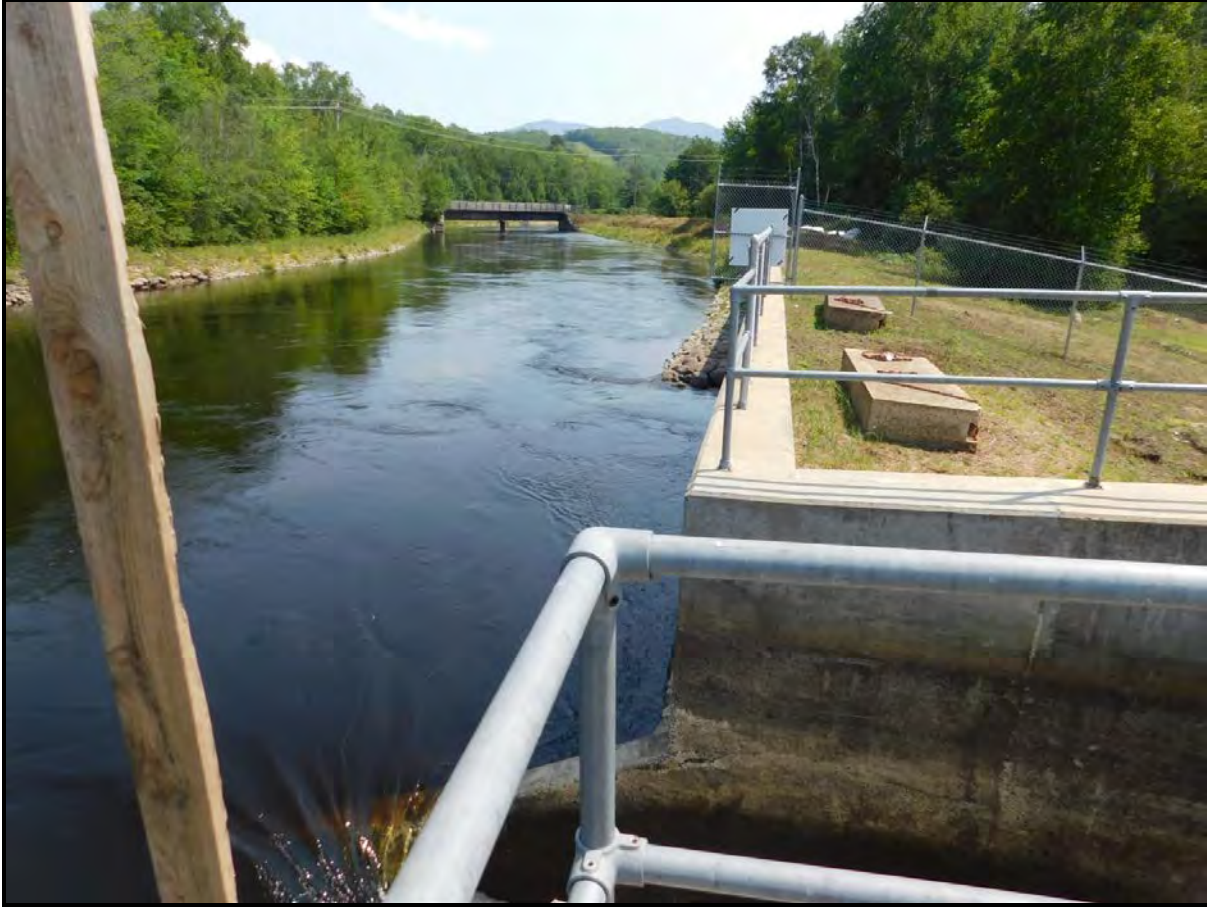
PHOTO 1-7 VIEW OF UPPER GORHAM PROJECT POWER CANAL AND ENTRANCE TO MINIMUM FLOW STRUCTURE.
