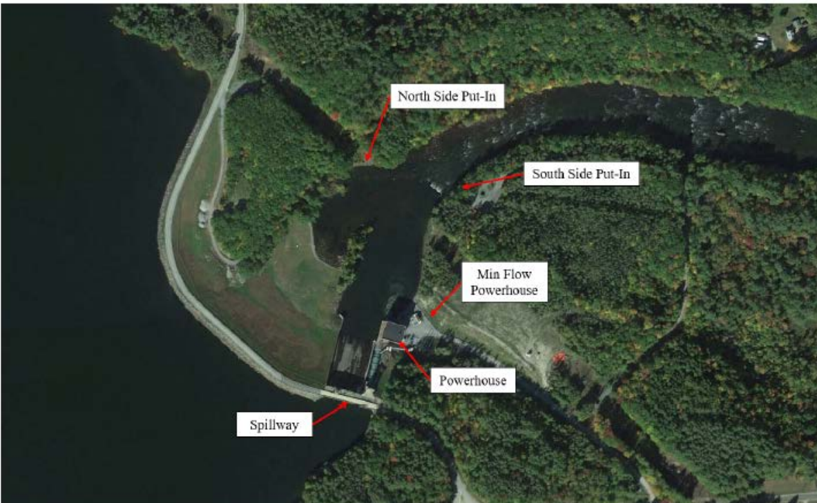
Figure 2 – Stewarts Bridge Hydroelectric Facility
