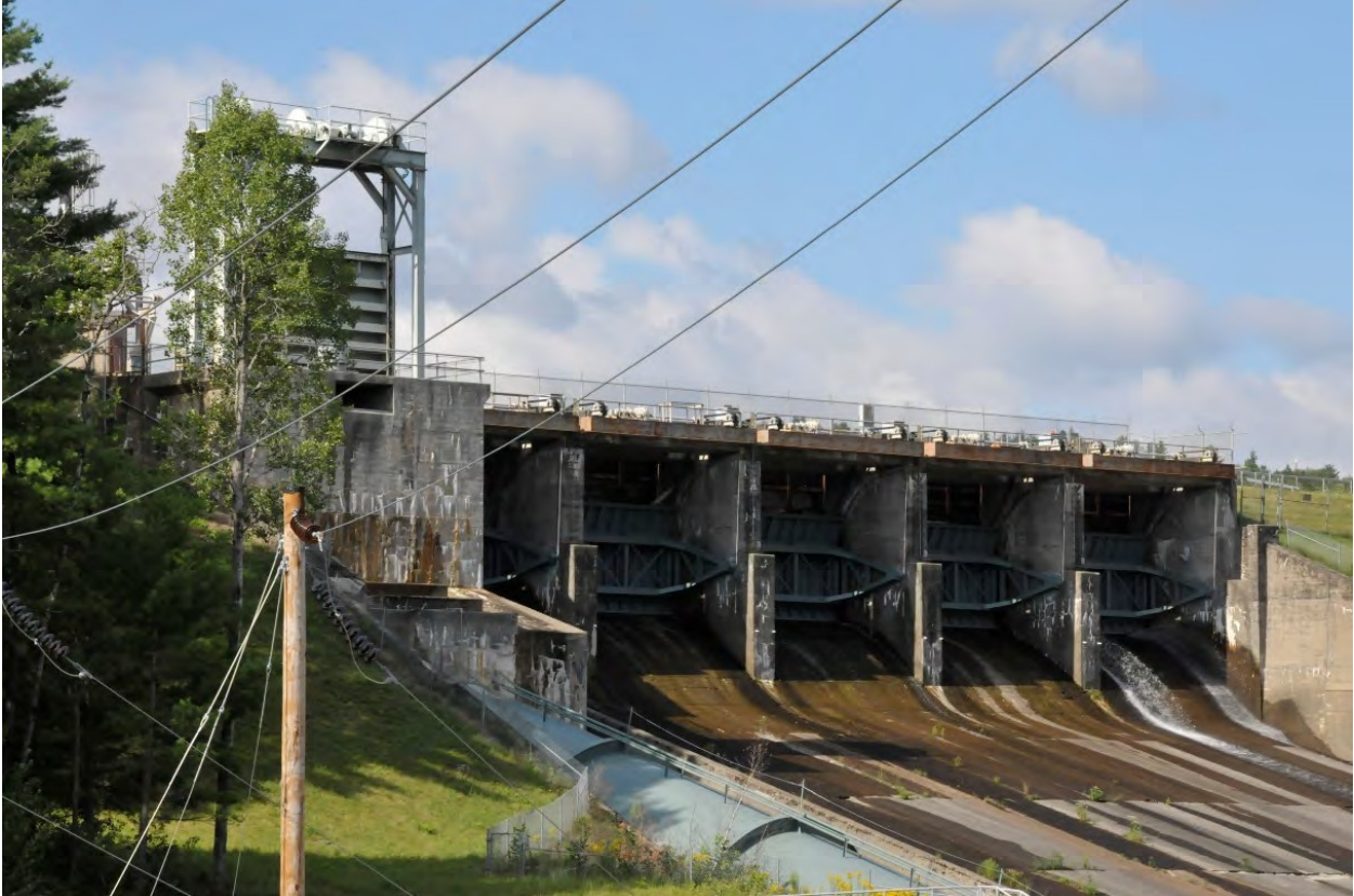
Figure 3 – Stewarts Bridge Dam, Spillway, and Penstock
