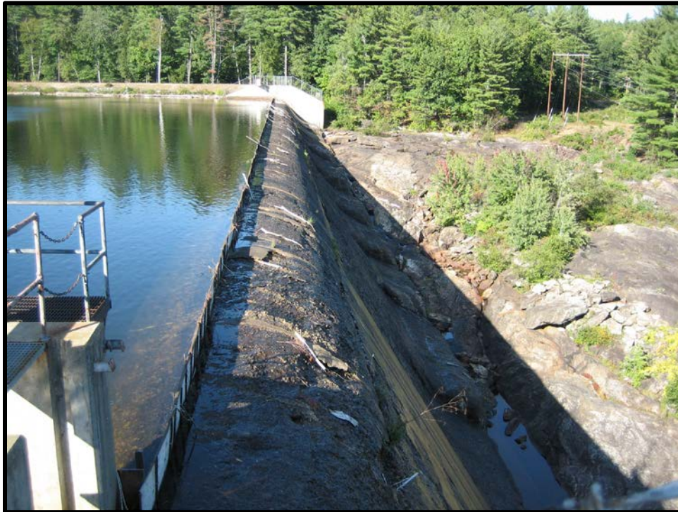
PHOTO 5-5 CREST OF THE OGEE SPILLWAY VIEWED FROM GATED STRUCTURE
