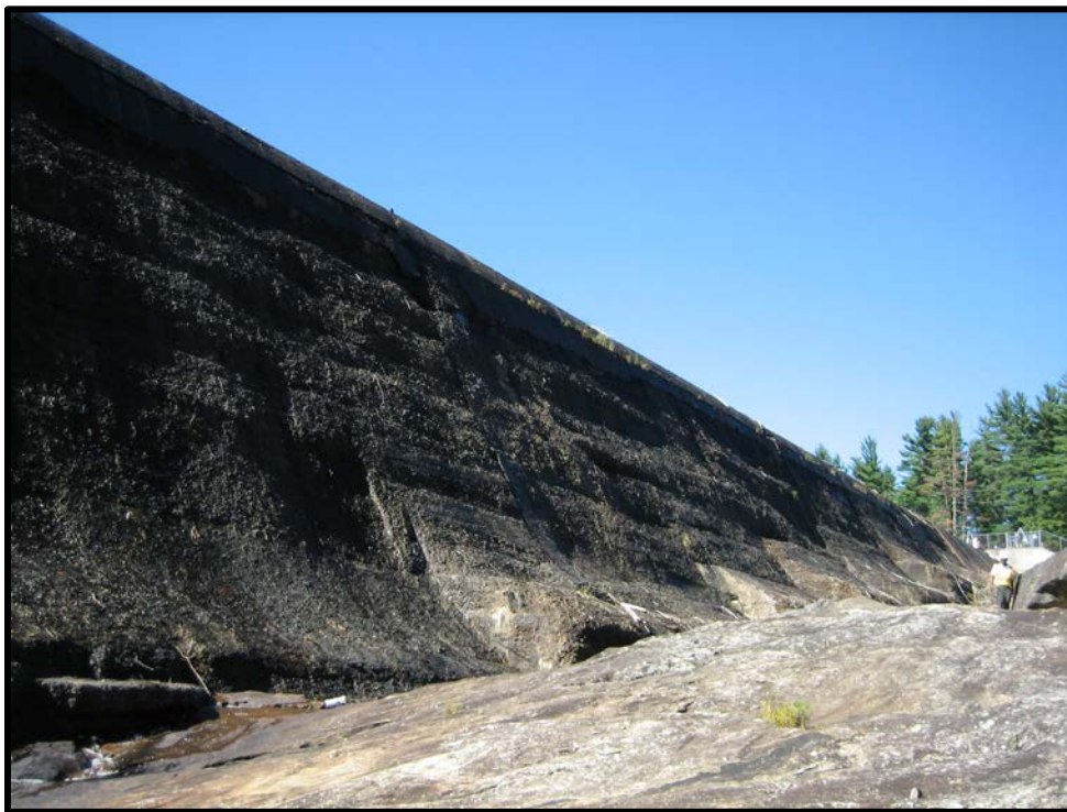
PHOTO 5-6 DOWNSTREAM TOE OF OGEE SPILLWAY VIEWED FROM BEDROCK AT DAM
