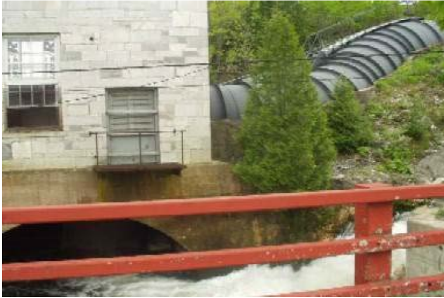
Photo 9 - Bifurcated Penstock to Powerhouse 1
