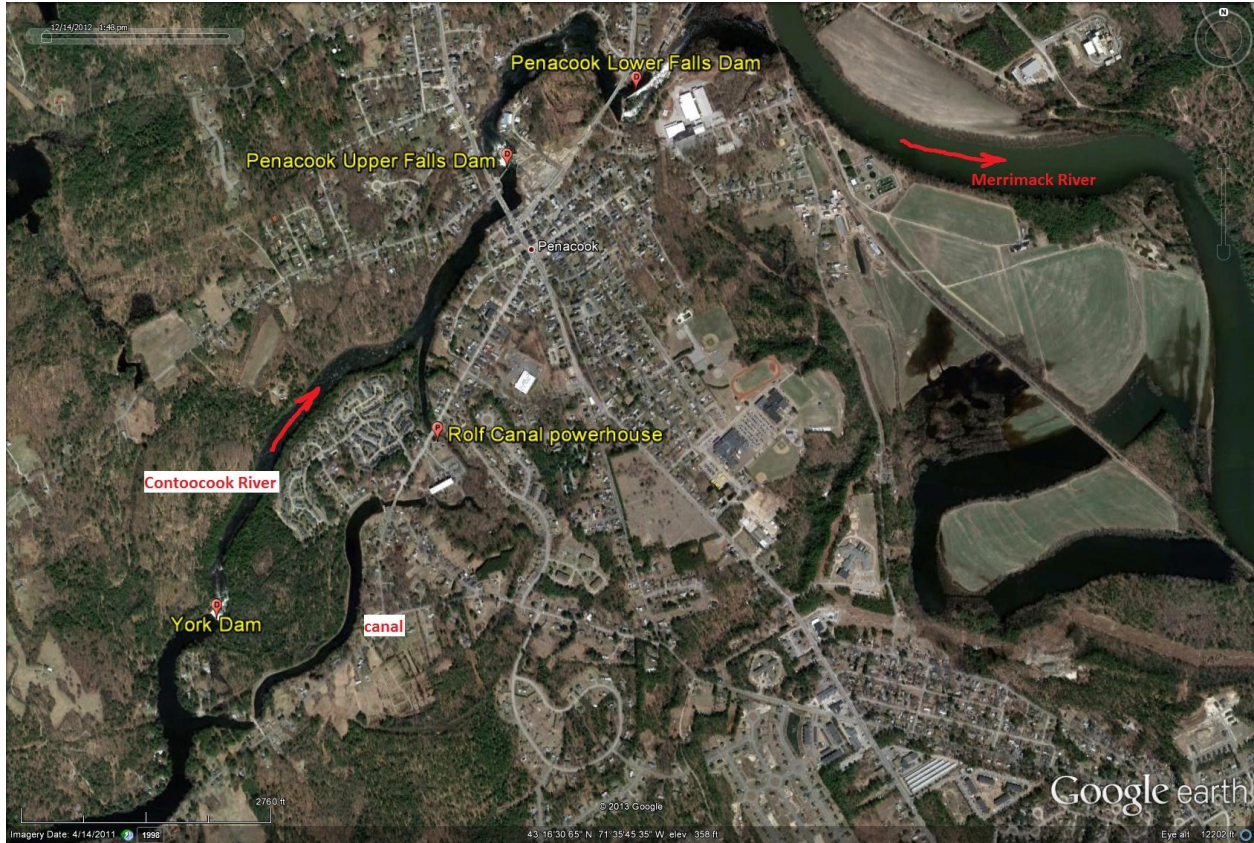
Figure 2. Rolfe Canal Hydroelectric Project and nearby dams.
