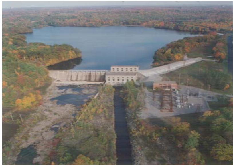
Photo 2 - Lighthouse Hill Dam and Powerhouse
