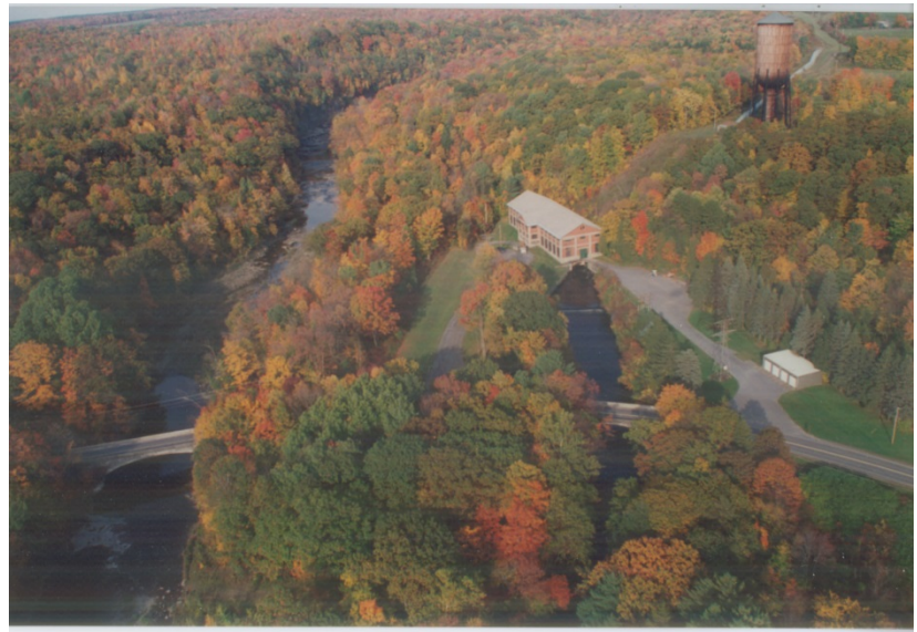
Photo 1 - Bennetts Bridge Surge Tank and Powerhouse
