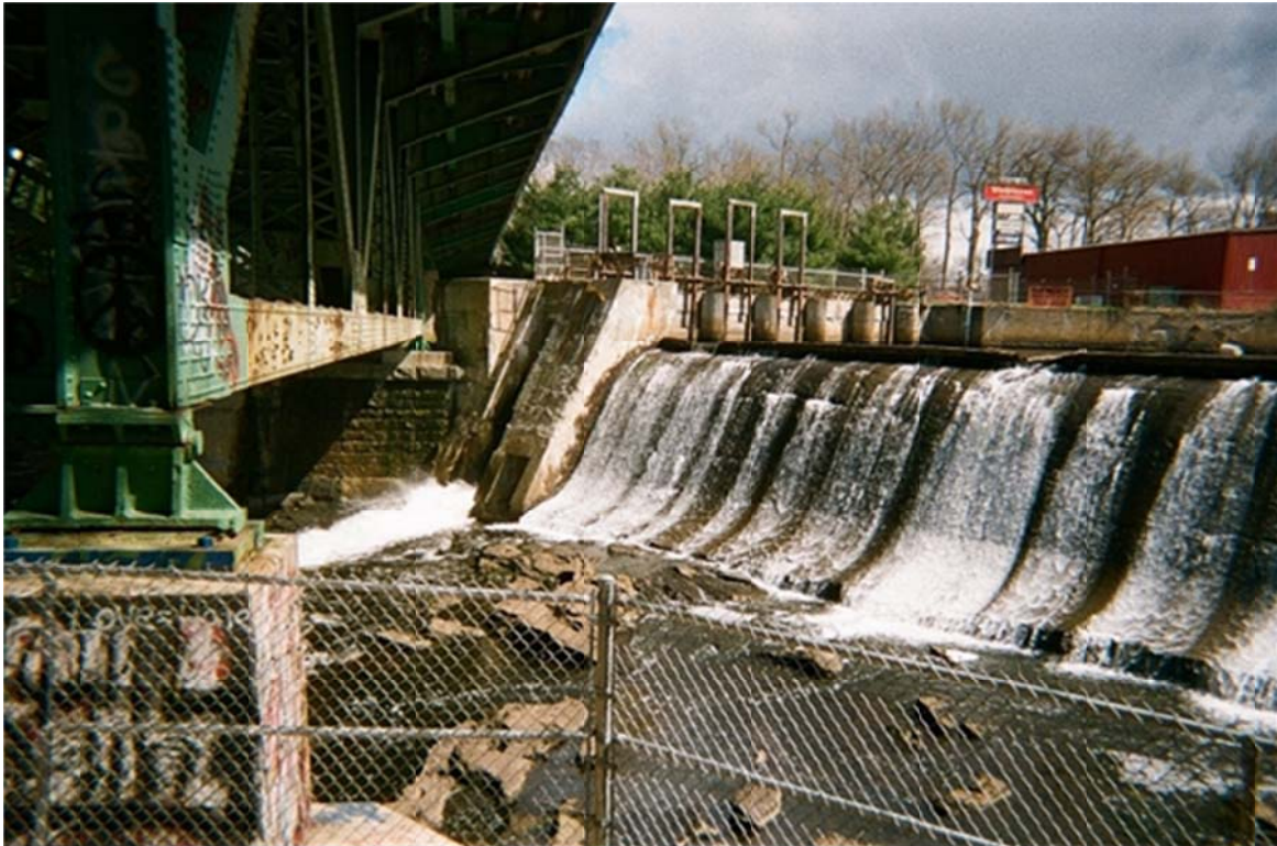
Putts Bridge Spillway, Skimming Gate and Head Gates
