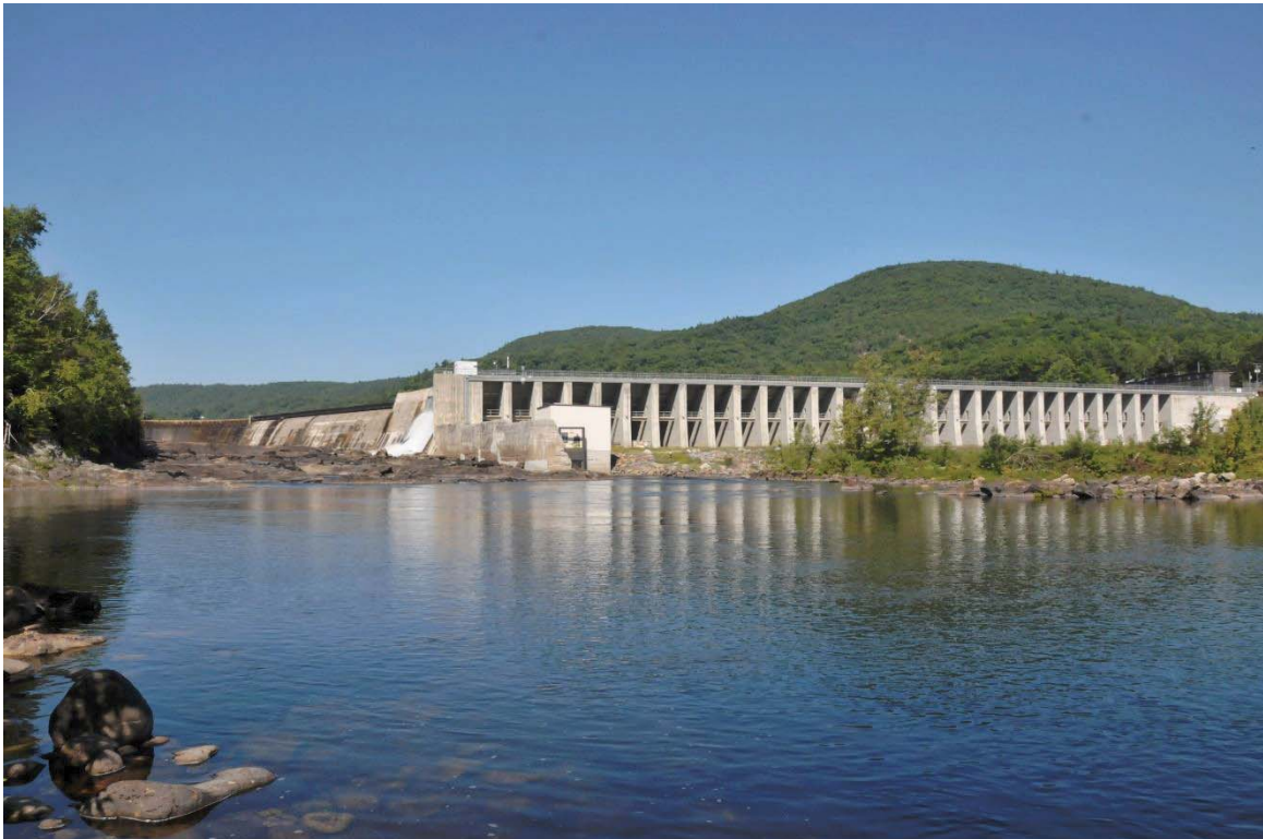
Bypass Reach and Minimum Flow Powerhouse
