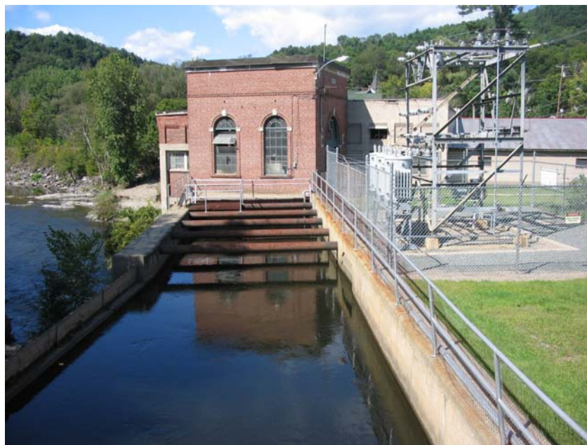
Figure 4 - Passumpsic Powerhouse and Power Canal
