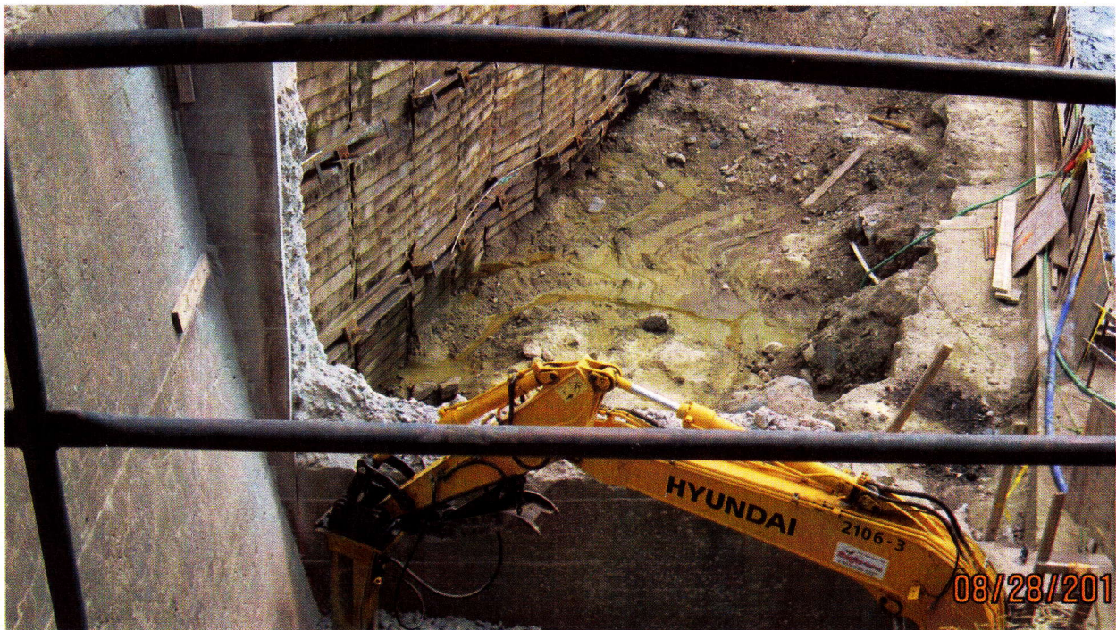
Photo 2. Beginning Demolition of Concrete Wall in Main Lift Area
