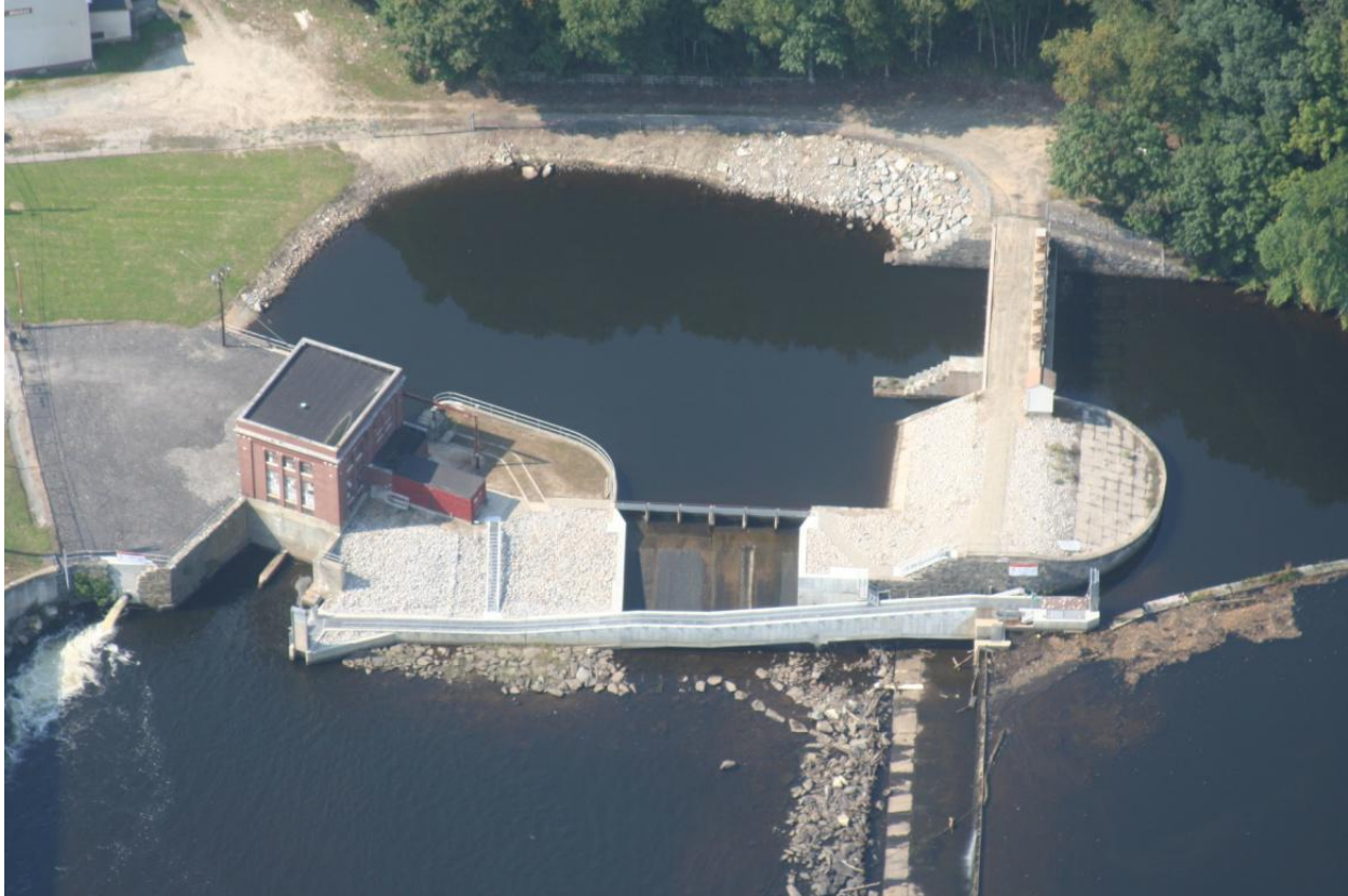
Figure 5. Aerial view of forebay and powerhouse. Denil fish ladder and downstream fish passage pipe (on left) shown.
