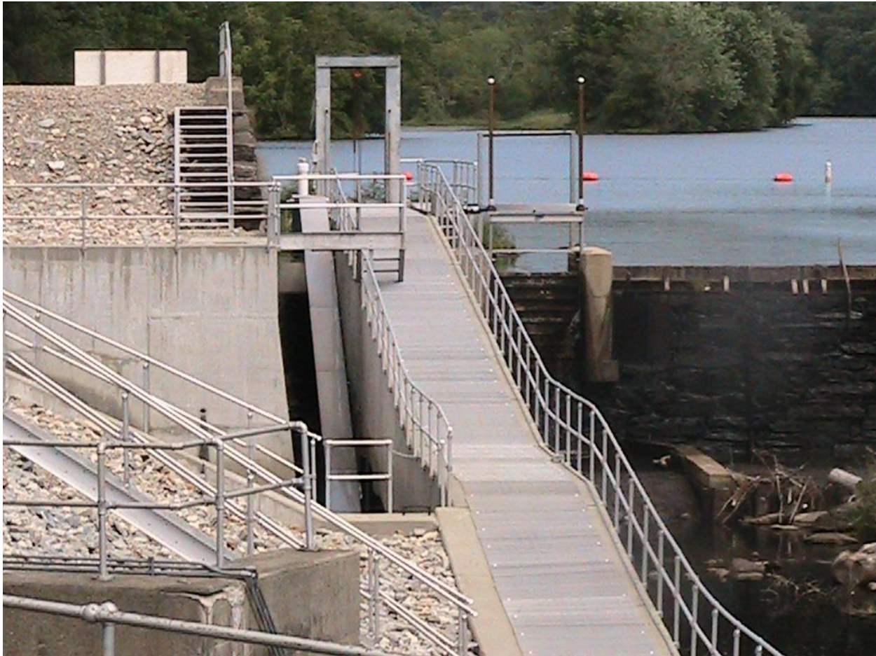
Figure 7. Eel pass is located between the dam abutment on left and the Denil ladder on right.
