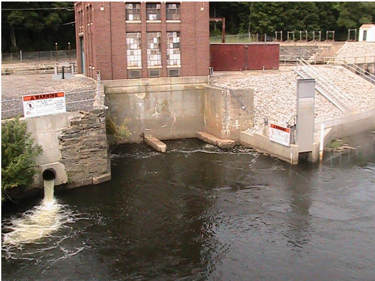
Figure 8. Power station with downstream migrant sluice pipe on left below tailrace; Denil ladder entrance on right.
