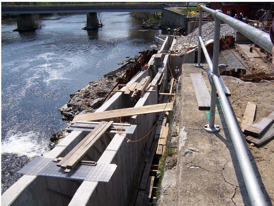
Photo No.2 - View of nearly completed concrete fish ladder looking downstream.
