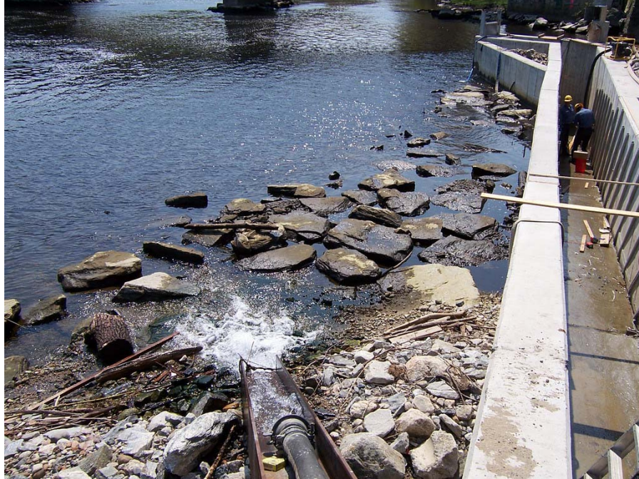
Photo No.3 - View of discharge of construction area leakage. No discernible turbidity was noted.
