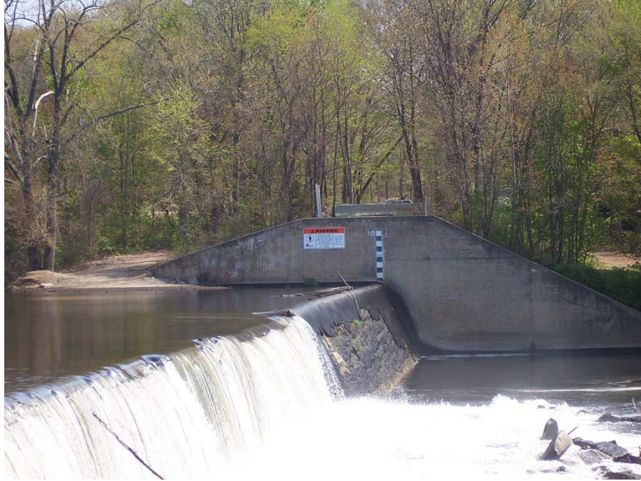
Photo No.7 - Upstream warning sign and staff gage on left dam abutment.
