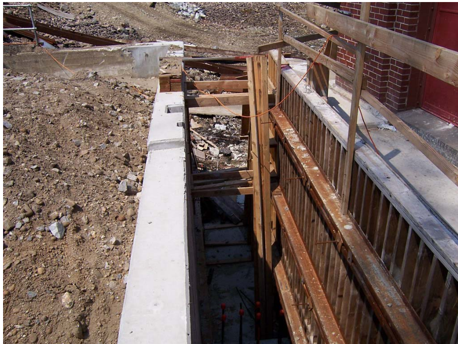
Photo No.4 - View of downstream passage facility nearing completion.
