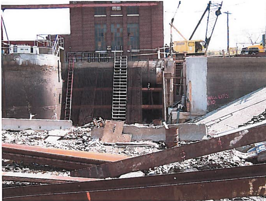
Photo No.5 - View of dewatered forebay area. Note downstream passage facility to right of trashracks.
