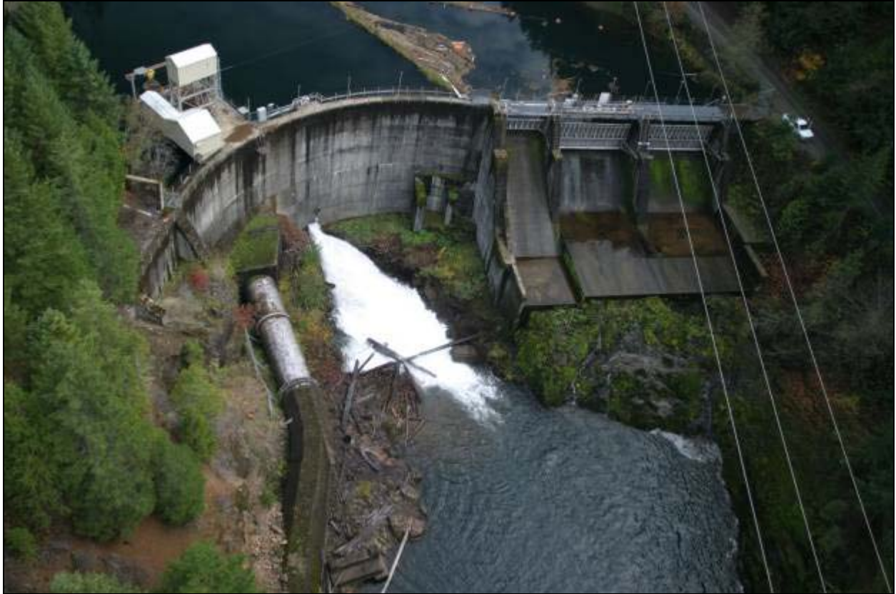
Figure 2.2-1 Soda Springs dam
