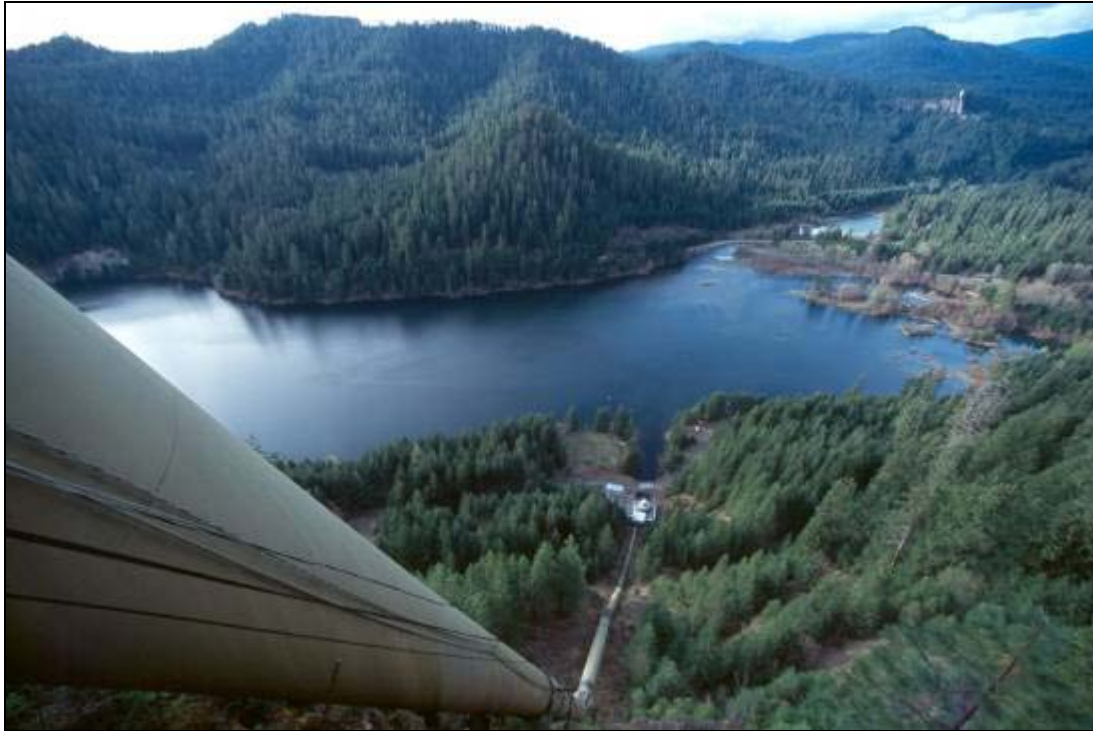
Figure 2.2-2 Clearwater No. 2 penstock and Toketee Lake
