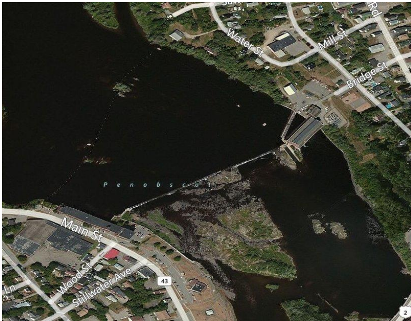
Milford Dam across the Penobscot River.
