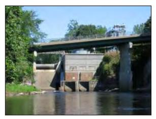
The powerhouse is integral with the dam and has an intake with 3-inch steel trashracks. There is one vertical Kaplan turbine generator with an installed capacity of 3.0 MW. Appropriate generator leads and transformers connect the Project to the interconnected transmission and distribution system at the switchyard located about 100 feet from the powerhouse.
