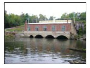
The powerhouse is located at the downstream end of the intake canal, and equipped with steel trashracks having a 1.75 inch clear spacing. Three Francis turbine units provide a total installed capacity of 2.25 MW. Appropriate generator leads and transformers connect the Project to the interconnected transmission/distribution system at the switchyard located 100 feet east of the powerhouse.
