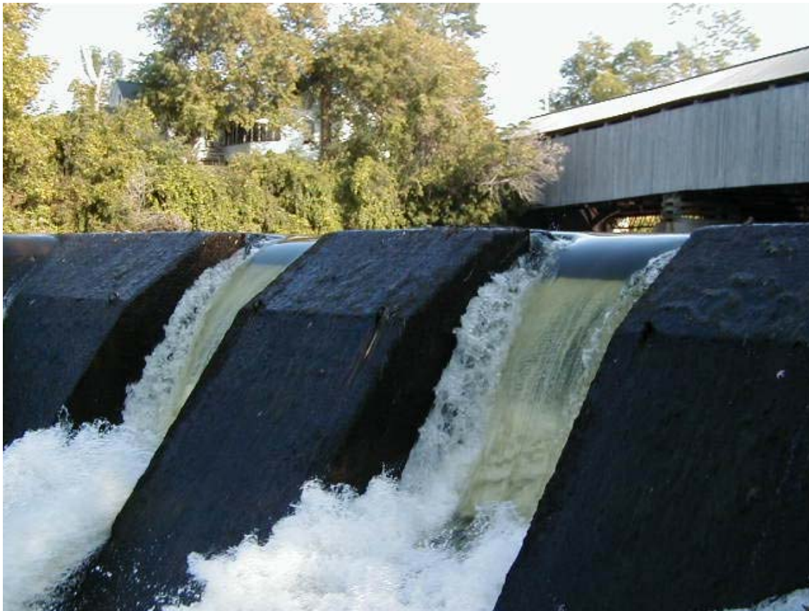
Photo 1. Sluice gates on West End of Dam with 2.6' of boards removed.
