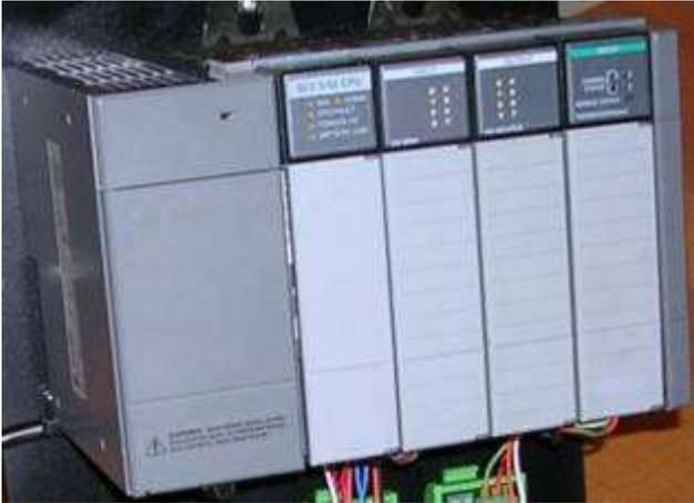
An Allen Bradley SLC-503 Programmable logic controller along with a pressure transducer in the forebay, continuously maintain the proper water elevation and will alert the Project operators of impending issues.
