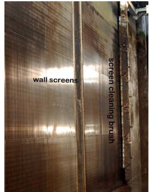
Photo 8. Wall screen and brush.
