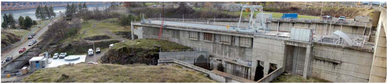
Photo 4. South side of the dewatering structure. The roof of the powerhouse is in the lower left corner of the picture.
