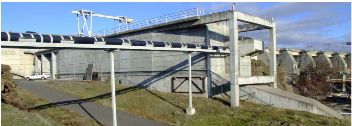
Photo 5. North side of dewatering structure and the bypass pipe that conveys fish to the tailrace.
