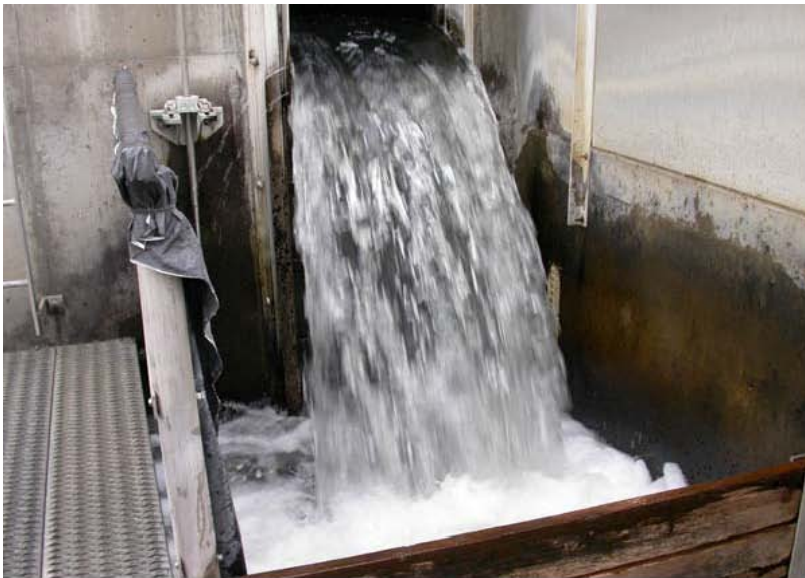
Photo 7. Weir discharge plunging into concrete basin.
