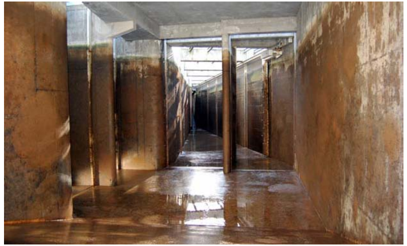
Photo 6. Interior view of the dewatering structure looking downstream. The diagonal wall screen is on the right.
