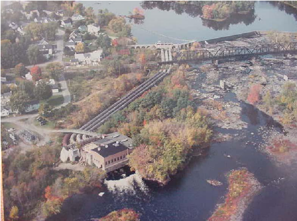
Note: Penstocks in photo were replaced during refurbishment
