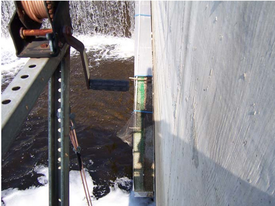
Photo No.6 - View of eel ladder, looking down from fish lift structure. Facility is operated by the CT Department of Environmental Protection during passage season.
