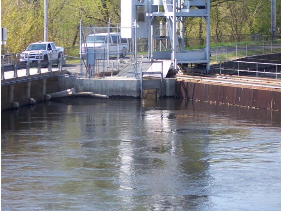
Photo No.7 - View of downstream fish passage entrance.
