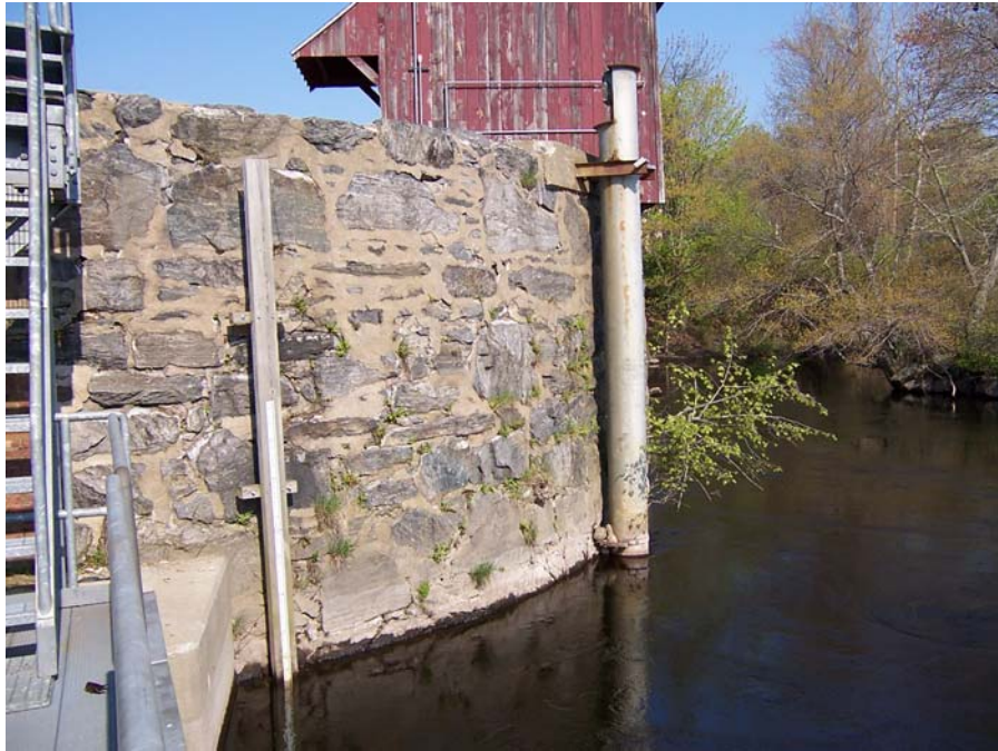
Photo No.1 - View of staff gage and pond level transducer at intake gatehouse.
