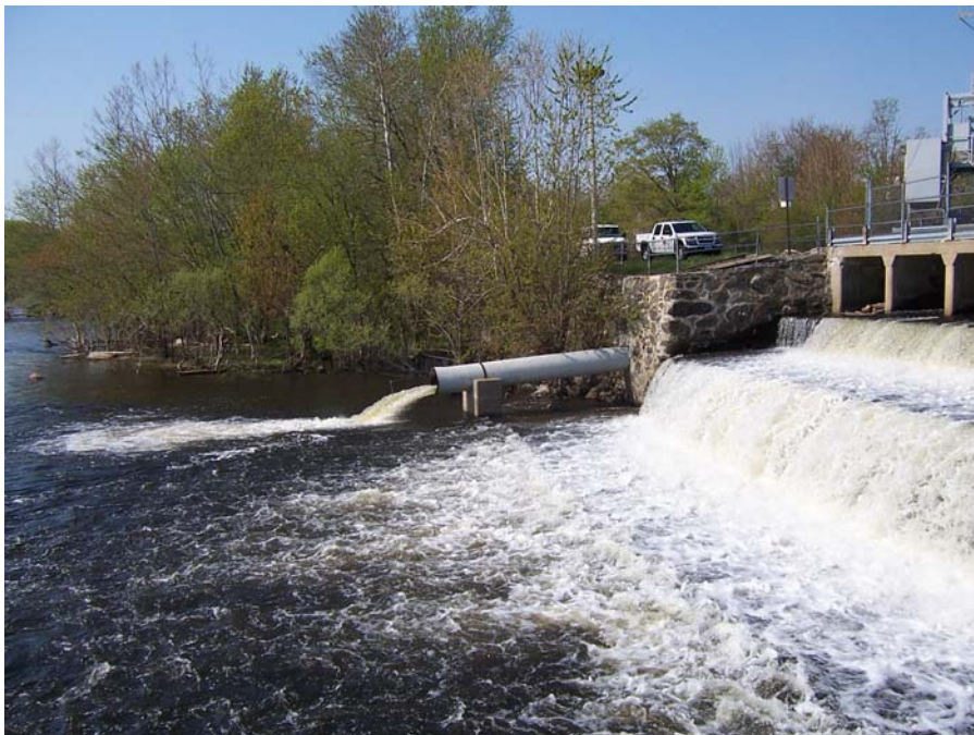
Photo No.8 - View of discharge from downstream fish passage facility.
