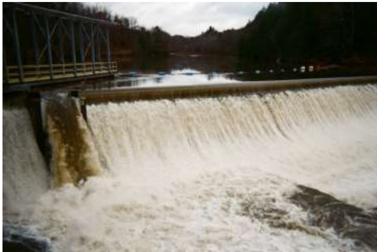
Minimum Flow Gate (left), Plunge Pool (bottom) and Dam (right)
