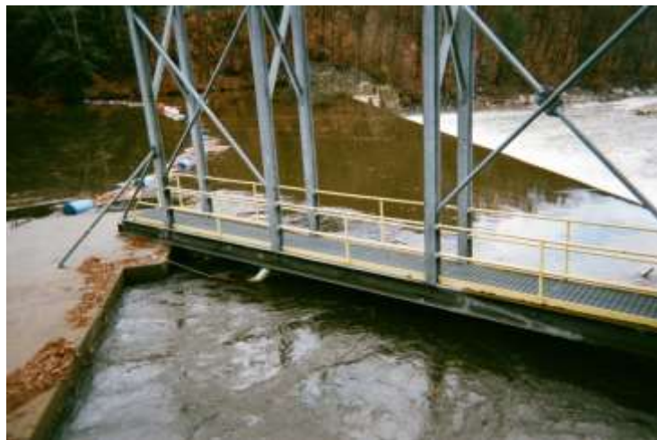
Walkway at Dam (Fish Louvers Attached)
